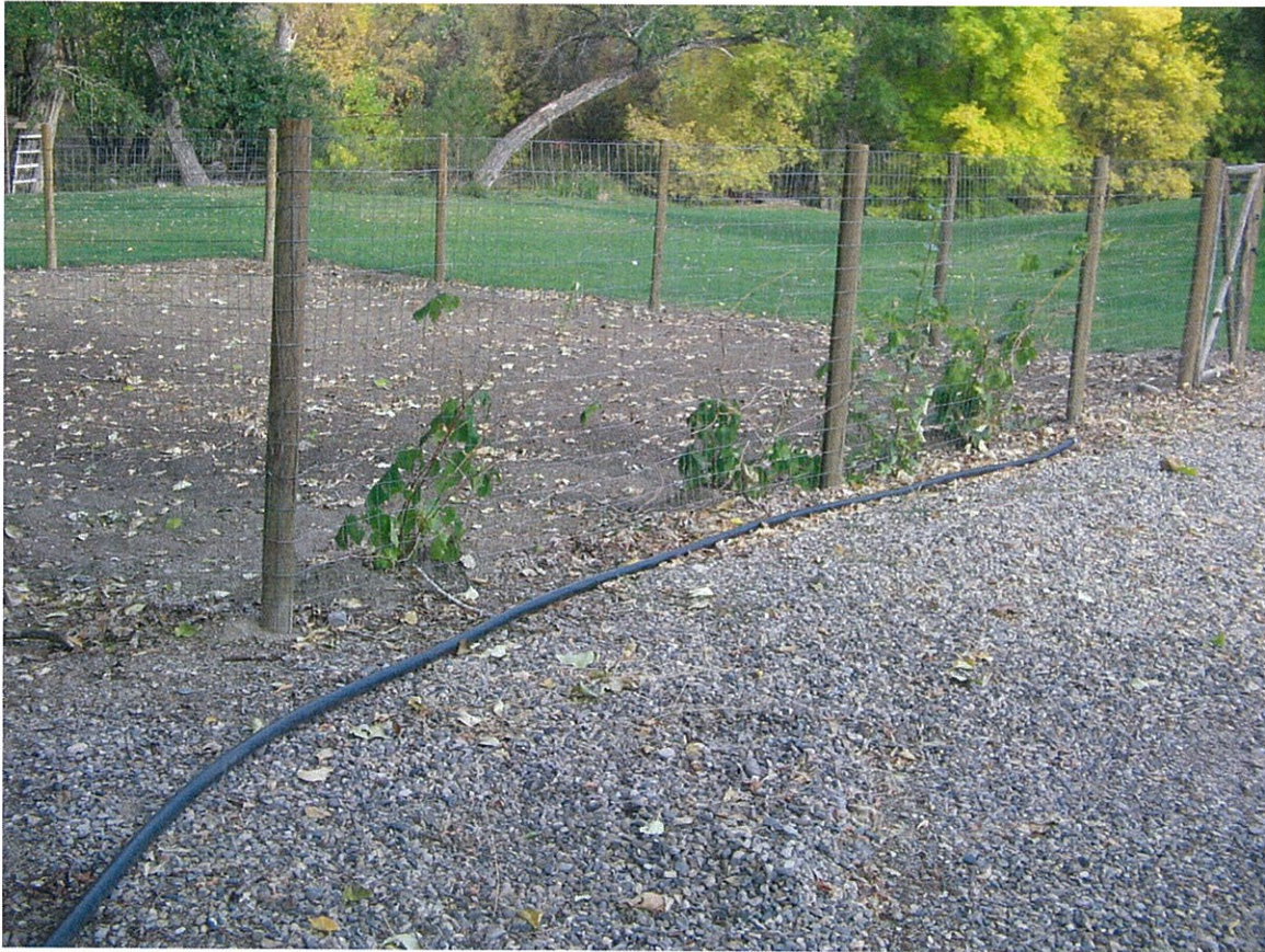
View of the 2" pipe entering the Engle property. The garden area can easily be seen, as can the irrigated lawn behind the house. The Jesse Creek channel is visible as the tree-covered area in the background.
