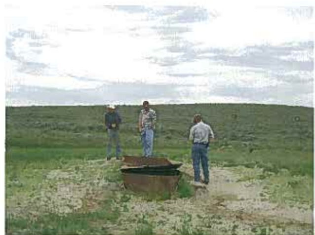
Figure 14. Stock Trough, located east of pivot, supplied by pipe described in Figure 12. Trough is 500 gallons and controlled by a float valve.
