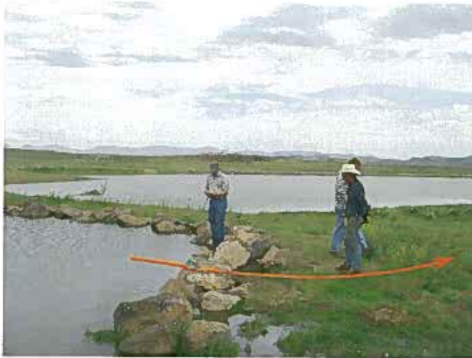
Figure 13. Location of buried pipe supplying stock trough. Pipe is 1 ½", plastic black pipe. Pipe is controlled by valve (currently underwater).
