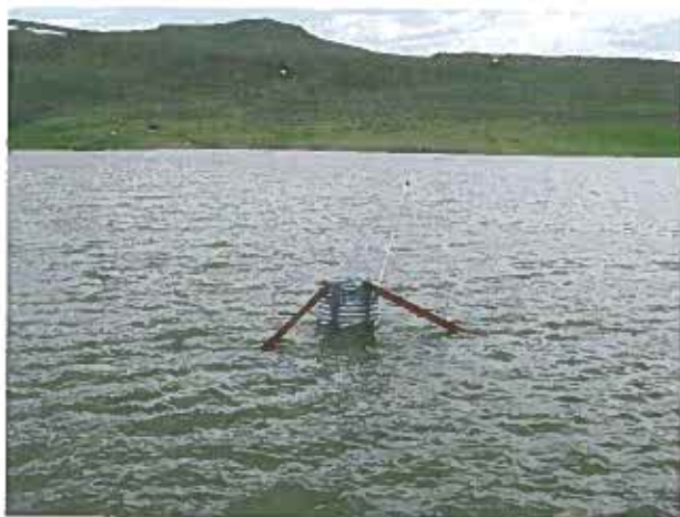
Figure 9. Control works (screw gate) located in the east pond for pivot.
