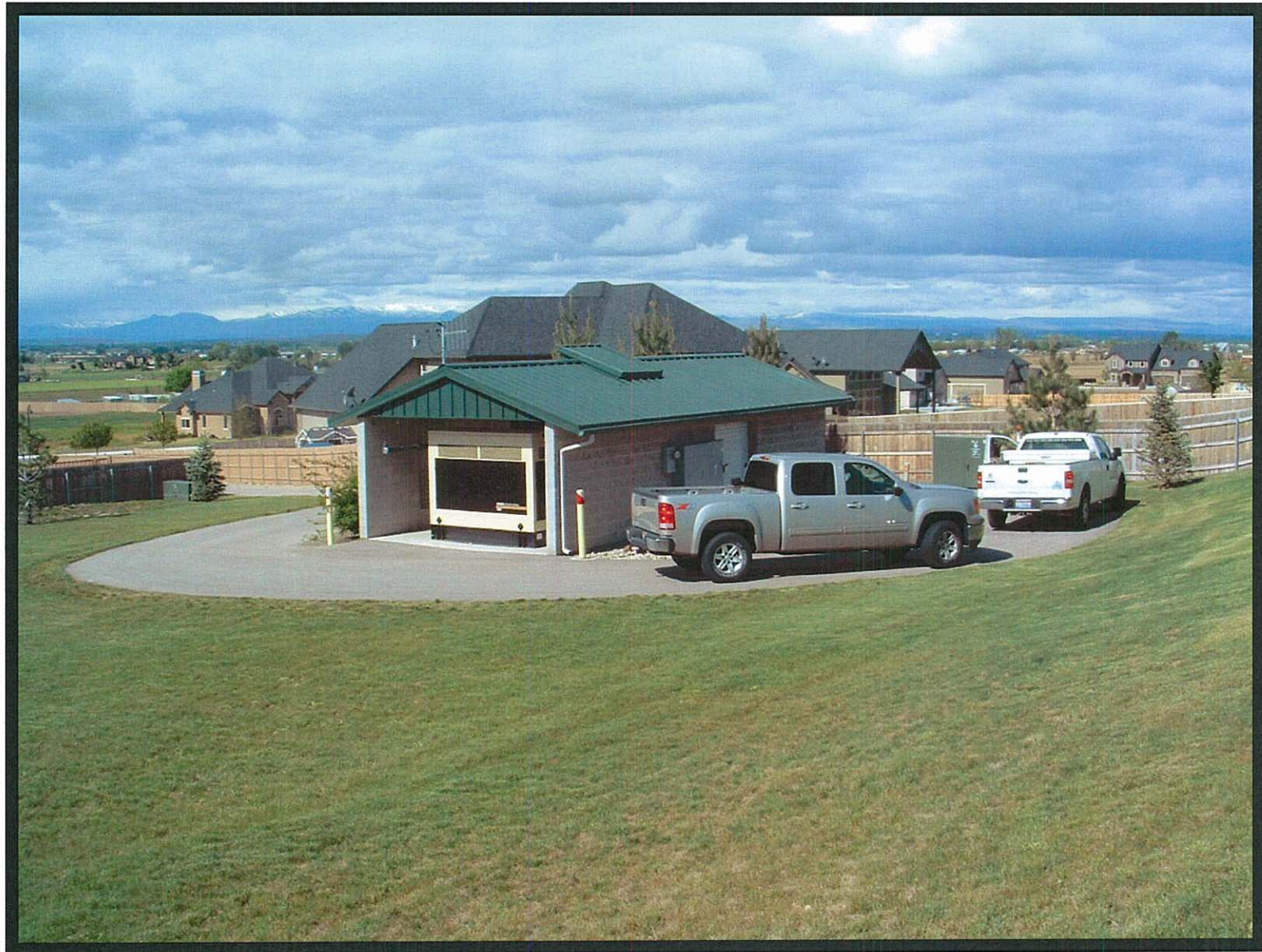
Well and Pump House, Lot 7, Block 1
