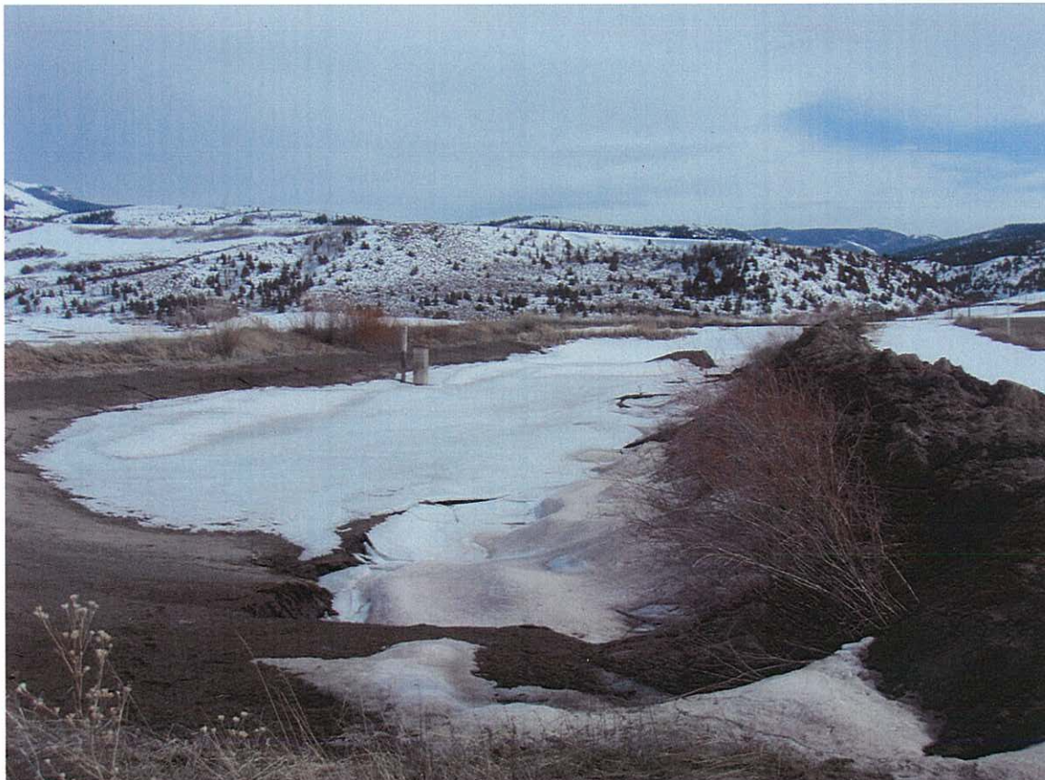
Photo 4 – View of the pond from the emergency spillway, looking south. The source ditch is located on the right (uphill) side; the embankment dam is located on the left (downhill) side.
