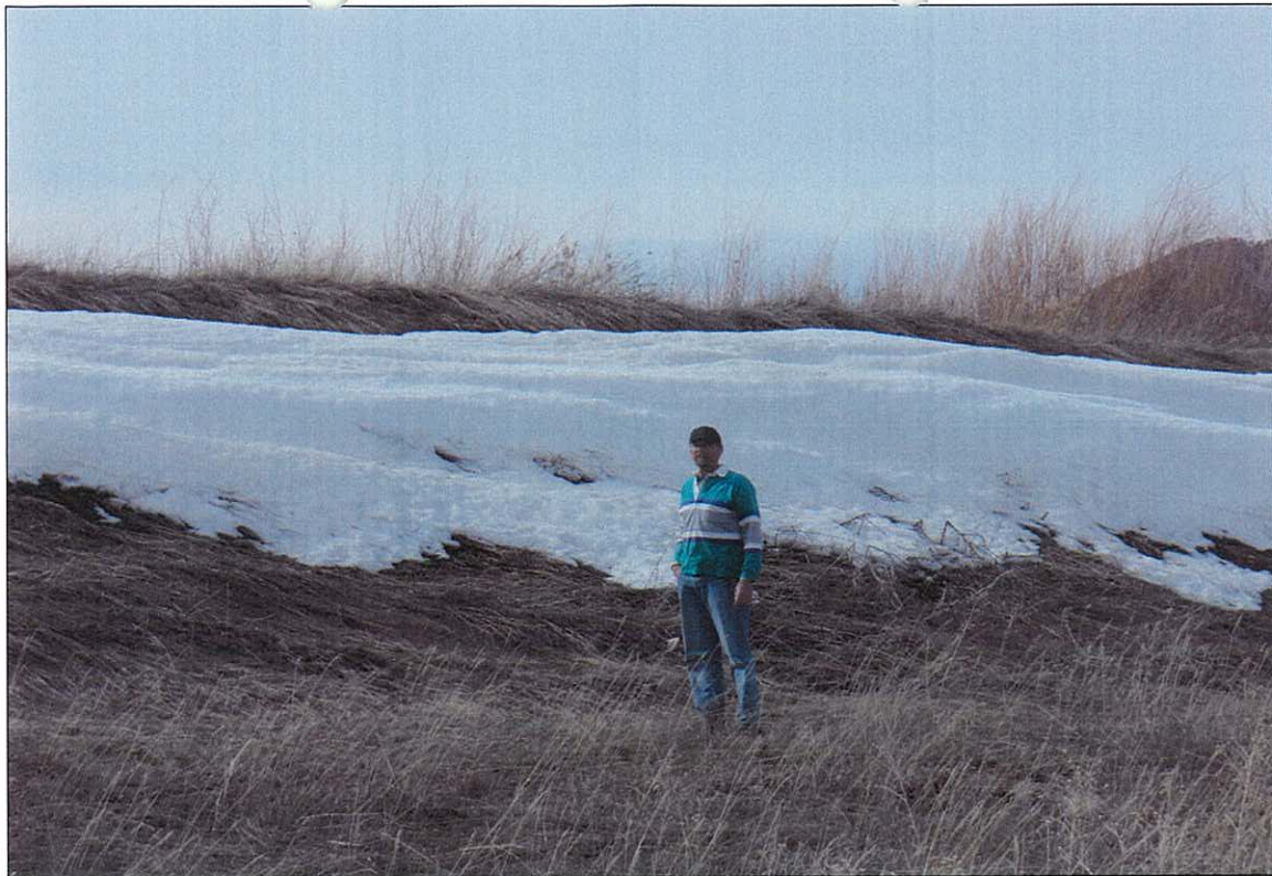
Photo 3 (4/4/08) – Downstream slope of dam near southeast corner
