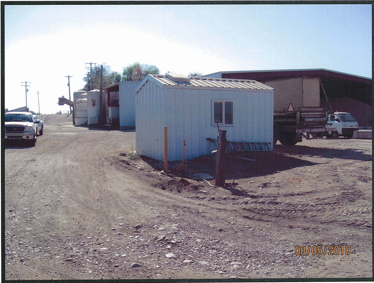
Well House for Wells 1 & 3
