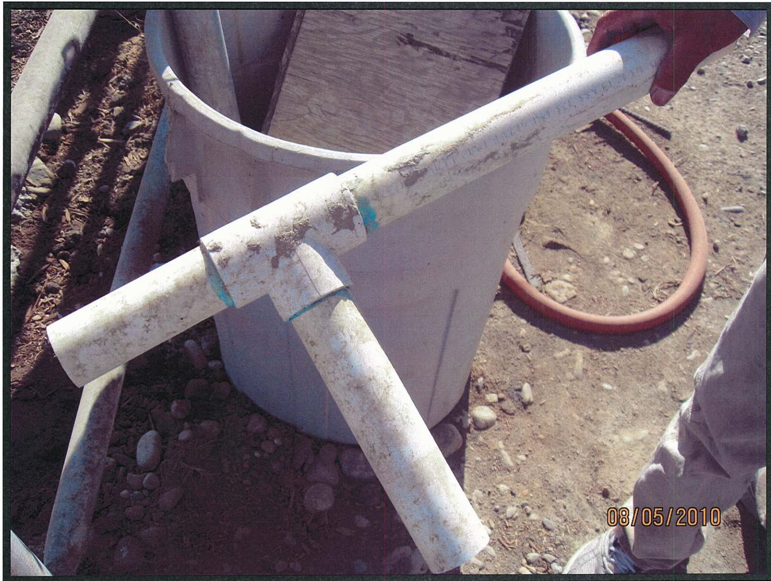
Sample of Buried Mainline (1.5-inch)
