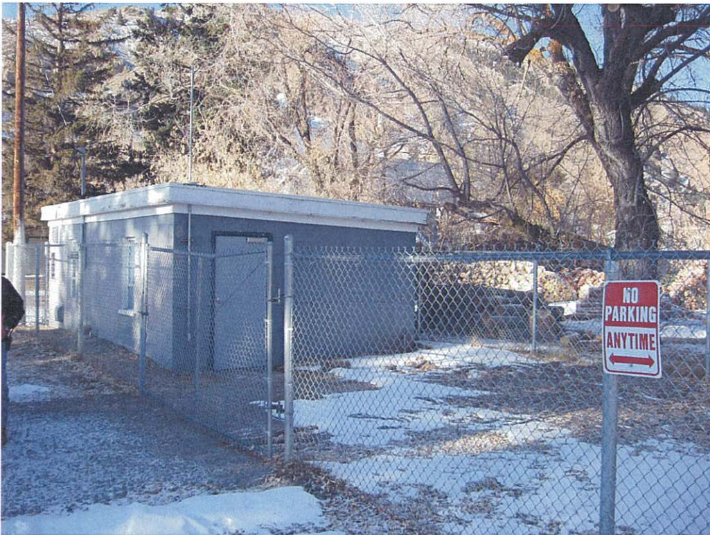
Figure 4: River Street pump house.
