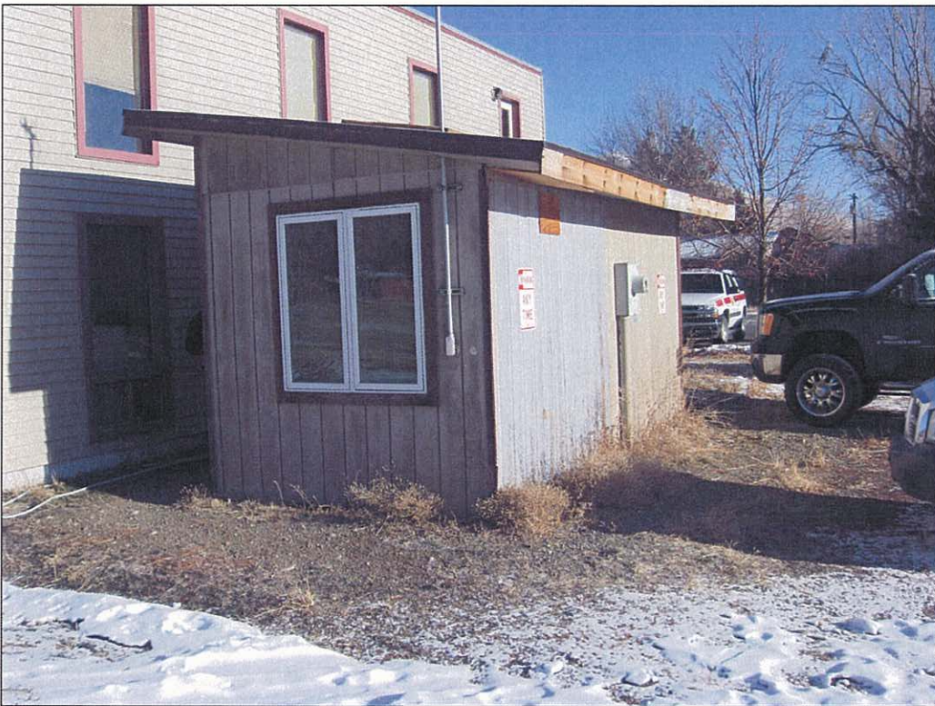
Figure 6: Third Ave pump house.
