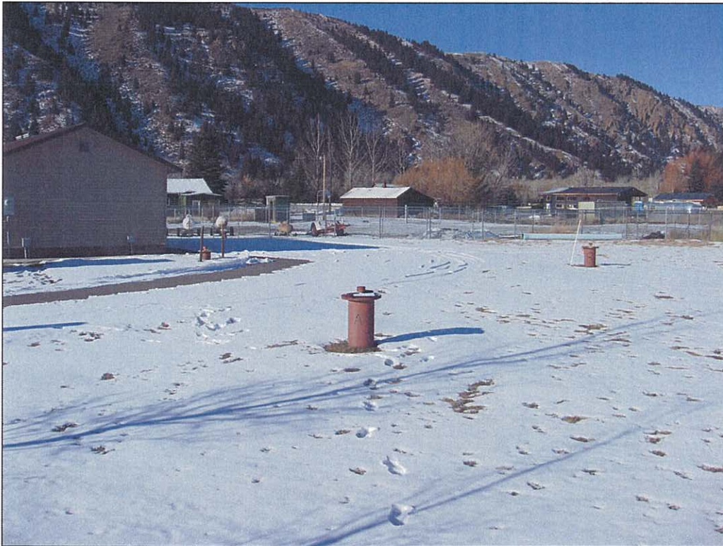
Figure 1: Northridge site well field with Well A in the foreground, Well B in the right background, and Well C in the left background. Pump house on photo left.
