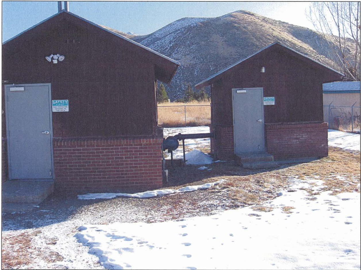
Figure 9: Woodside well house (right) and booster pump house (left).
