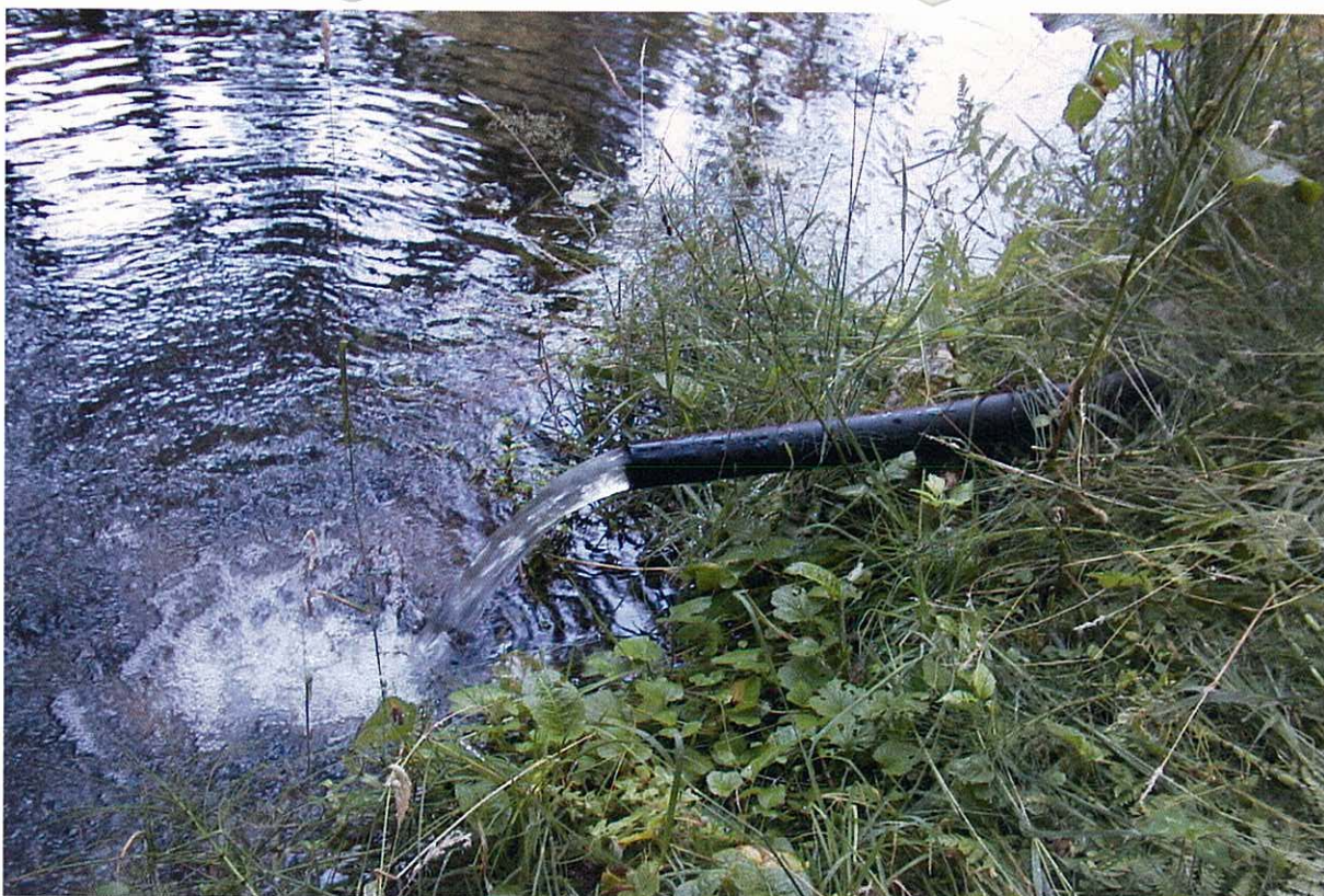
FIGURE 3: 2" outlet into upper pond.
