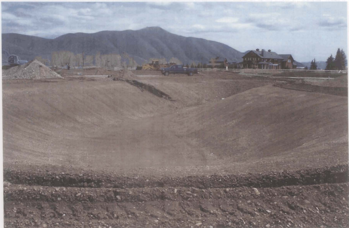
Tanner Pond Under Construction By J E Stanton May 2002
