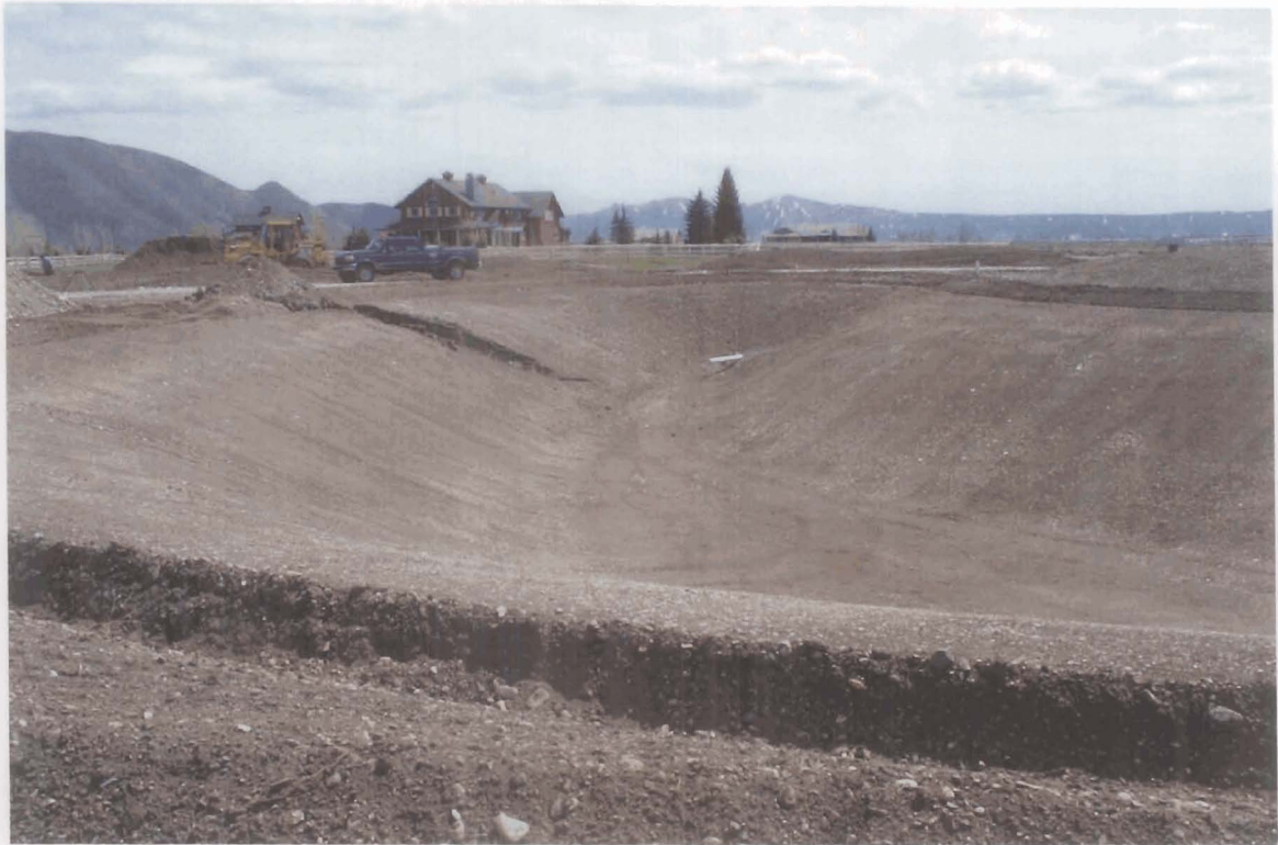
Tanner Pond Under Construction (Bloomfield Home In Background) By J E Stanton May 2002
