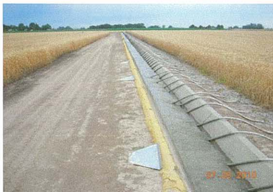
At concrete trapazoidal ditch, looking west. Siphons serve field to the north.
