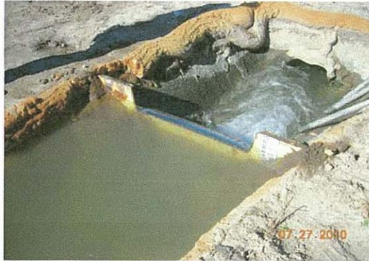
Temporary Cipolletti Weir at end of concrete ditch. Ground water only, no surface water at time of measurement
