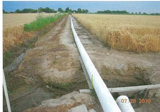
South boundary of property, looking west. 10-inch gated pipe to serve field to the north. Drain ditch in foreground flows to the right (north)
