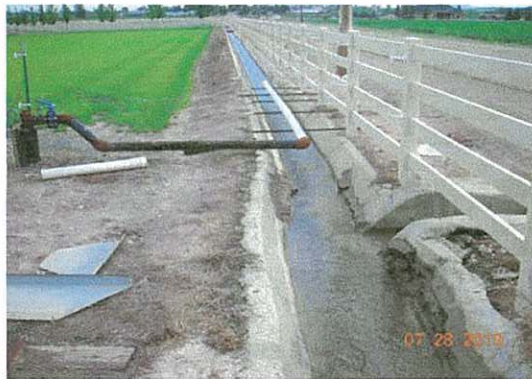
At SE corner of property looking north along Ridgewood Rd. Nampa Meridian Irrig. Dist. Water entering ditch from east and south Photo taken day after well test.
