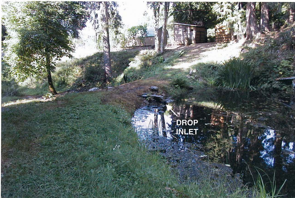
FIGURE 6: Second dam impounding middle pond, downstream is to the left.
