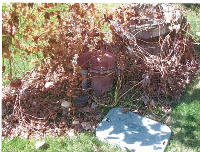
Figure 5. Well and irrigation control works located adjacent to the most southern residential structure.
