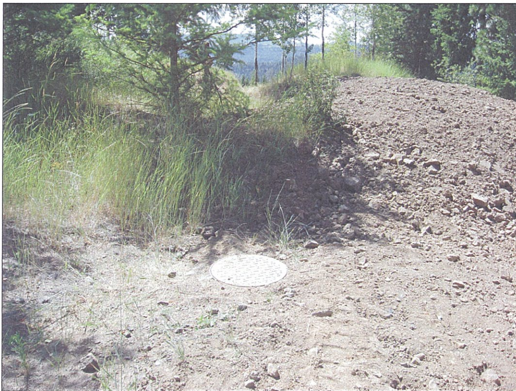
Photo 4: Access to valve and flowmeter vault is through this manhole, located in NENE Section 17.
