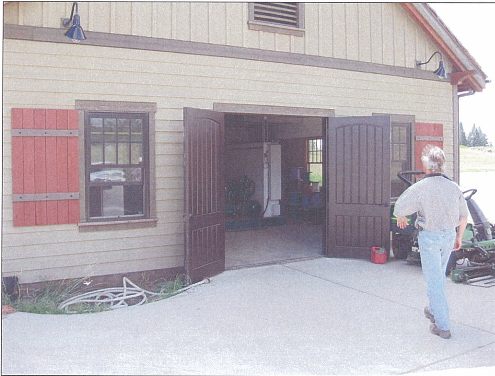
Photo 11: Black Rock North pump station building.
