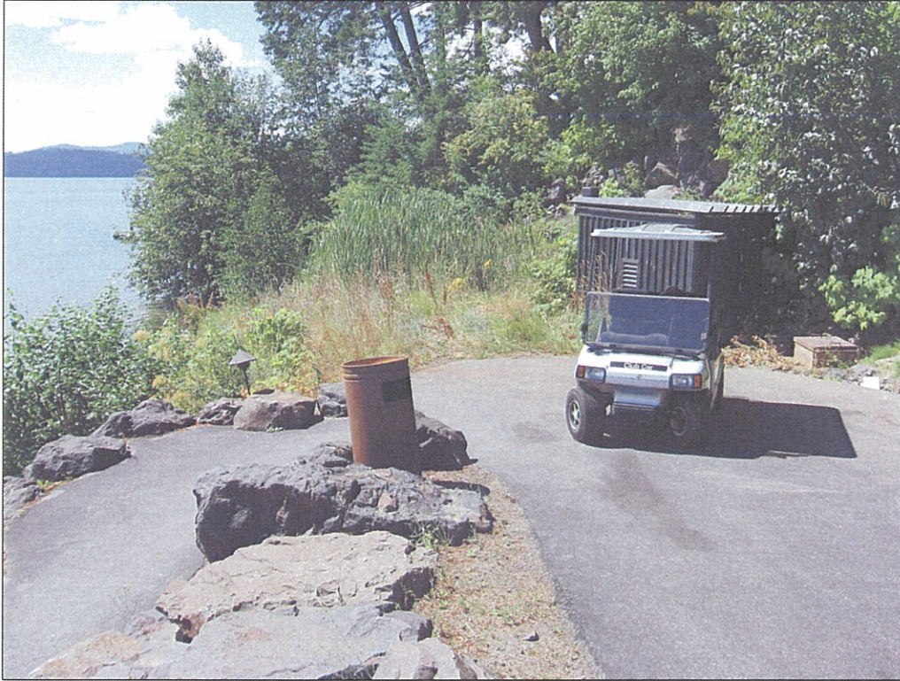
Photo 1: Point of Diversion. Intake is in lake to photo left. Power transformer, panels, and VFDs are located in the structure behind the Club Car. Access to the vault is at photo right.
