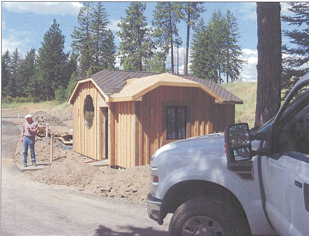
Photo 5: Potable municipal water supply booster station for 95-9055 is located near the valve and flowmeter vault.
