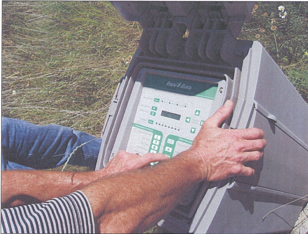
Photo 17: Controller for golf course irrigation system.
