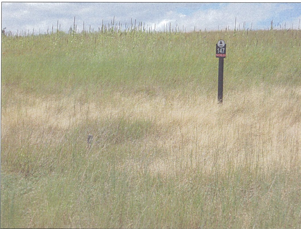
Photo 20: Wooden stake in photo lower left marks the location of water services stubbed in to residential lots where homes are not yet constructed.
