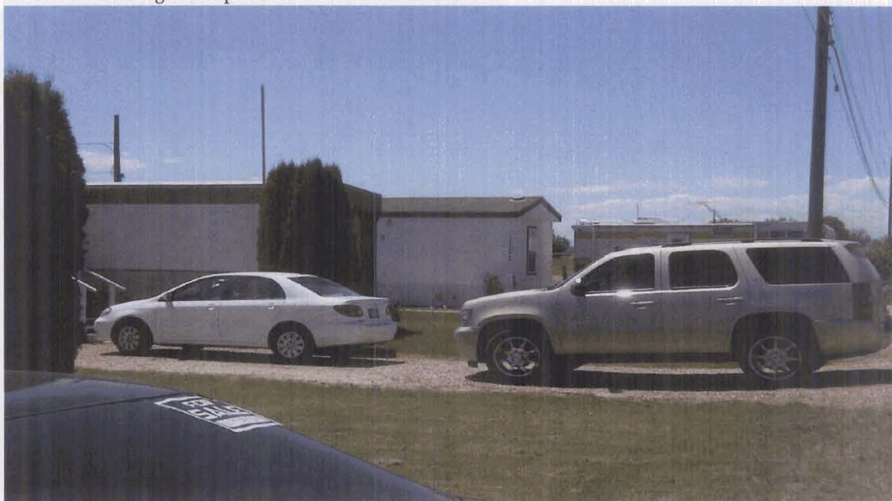
Trailer park looking east.
