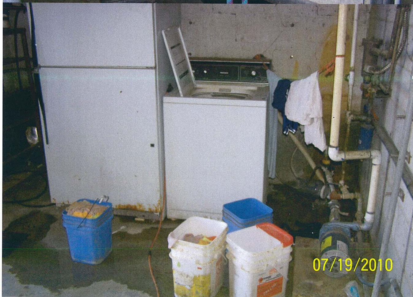
Washer Dryer Room, inside the Milking Barn
