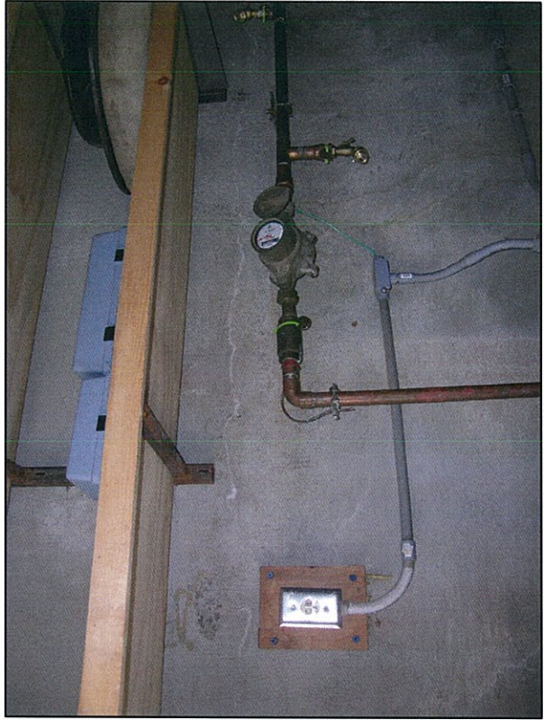
Pic. 8 – Well No. 3 Sensus 3/4" SRII totaling meter.
