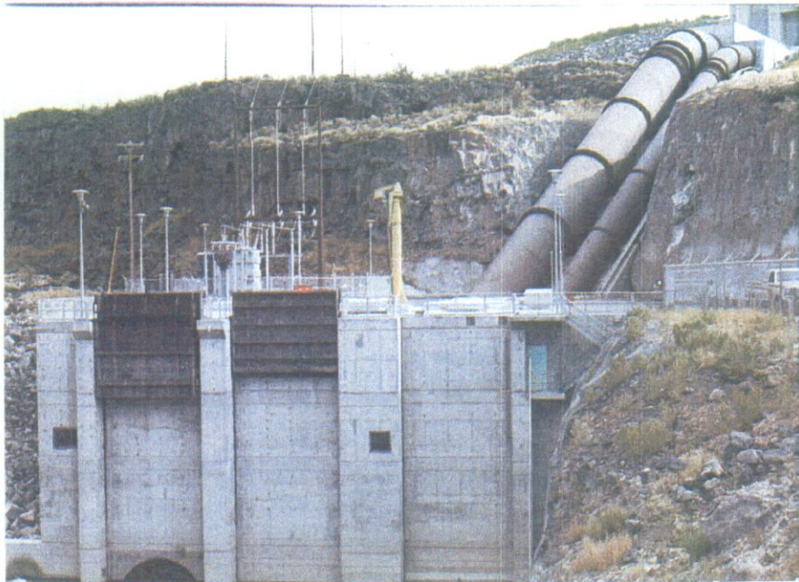
Milner Main Power House
