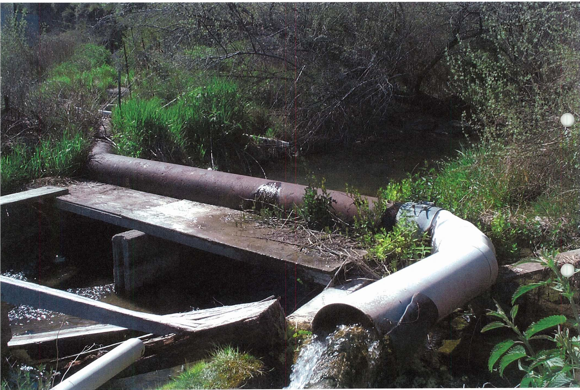
47-7659 Pipeline From Upper Raceways Across Slaughterhouse Creek Looking SSW 5-19-09. Ru T Stanton
