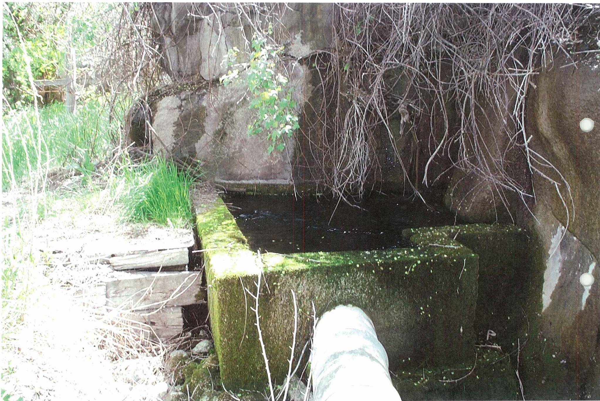
47-7659 Diversion Works Looking SE
