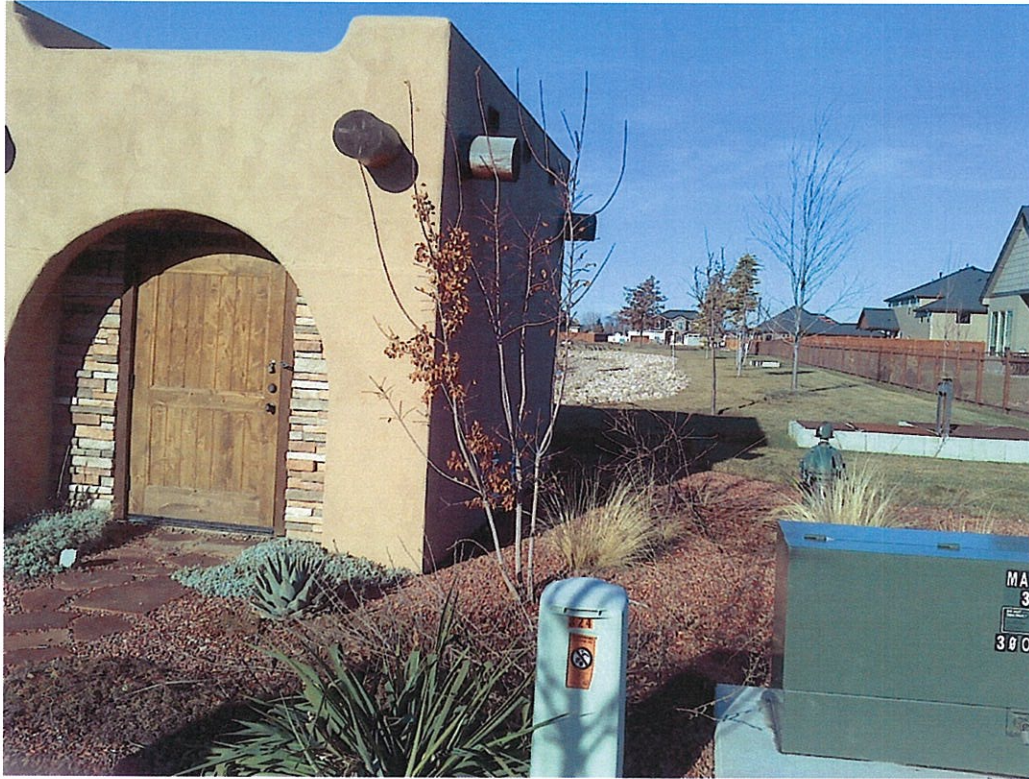
Photo 5: Pump house is on left, well head - middle right, irrigation box for surface water – behind well head, pond is directly behind pump house; looking north
