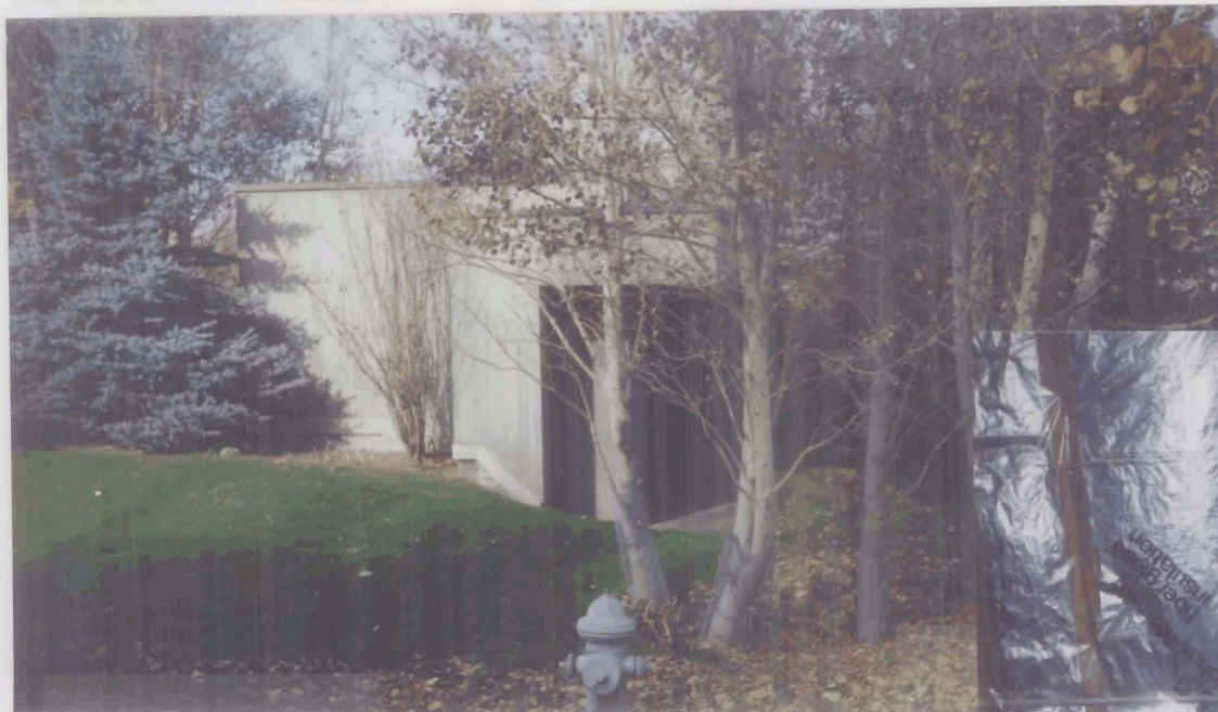
Pumphouse, Lot 6 Riverwoods Subd.
