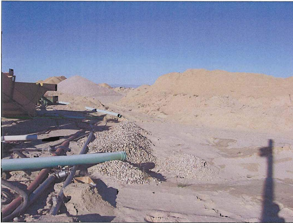
Photo 5: Place of use is at gravel pit.
