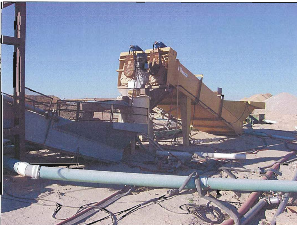
Photo 6: Gravel washing equipment.
