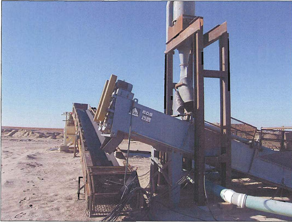
Photo 7: Gravel washing equipment.
