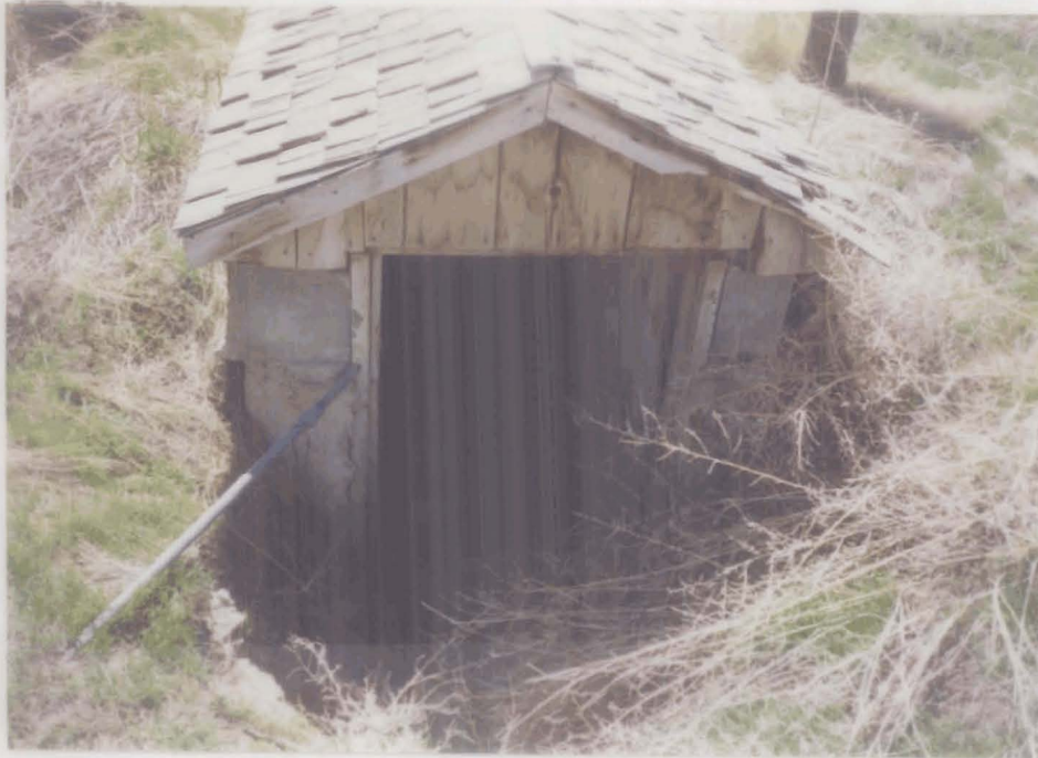
This is the well house for well #2
