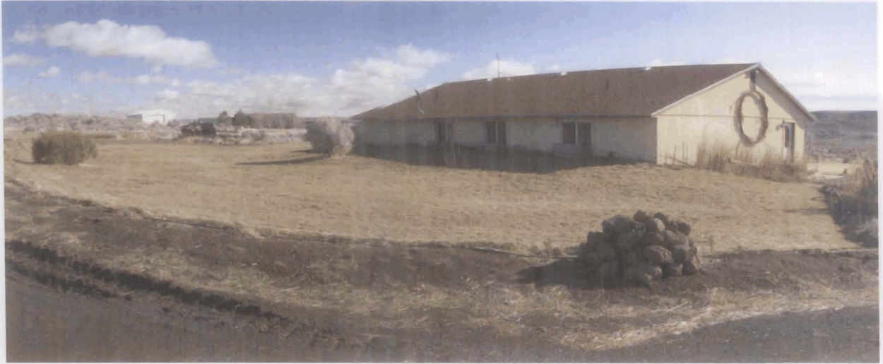
Figure 1: Front Yard and house of property.
