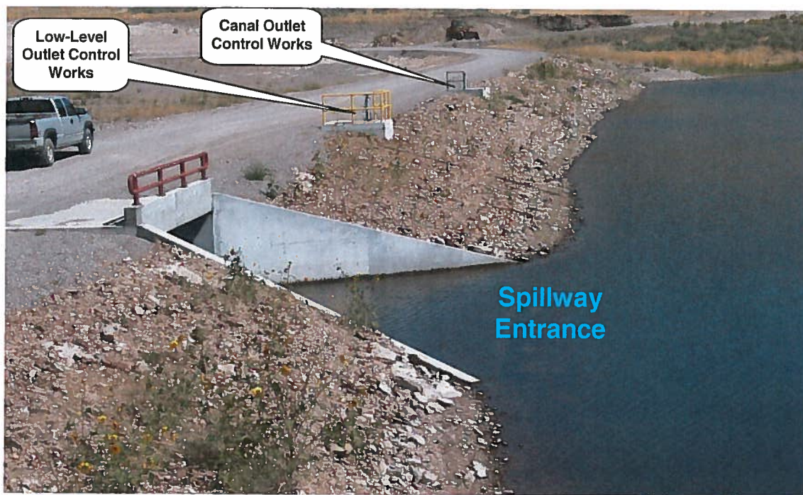
ABOVE: View of the dam crest and the upstream slope of the dam from near the left (west) end of the dam with the locations of various points of interest indicated.
