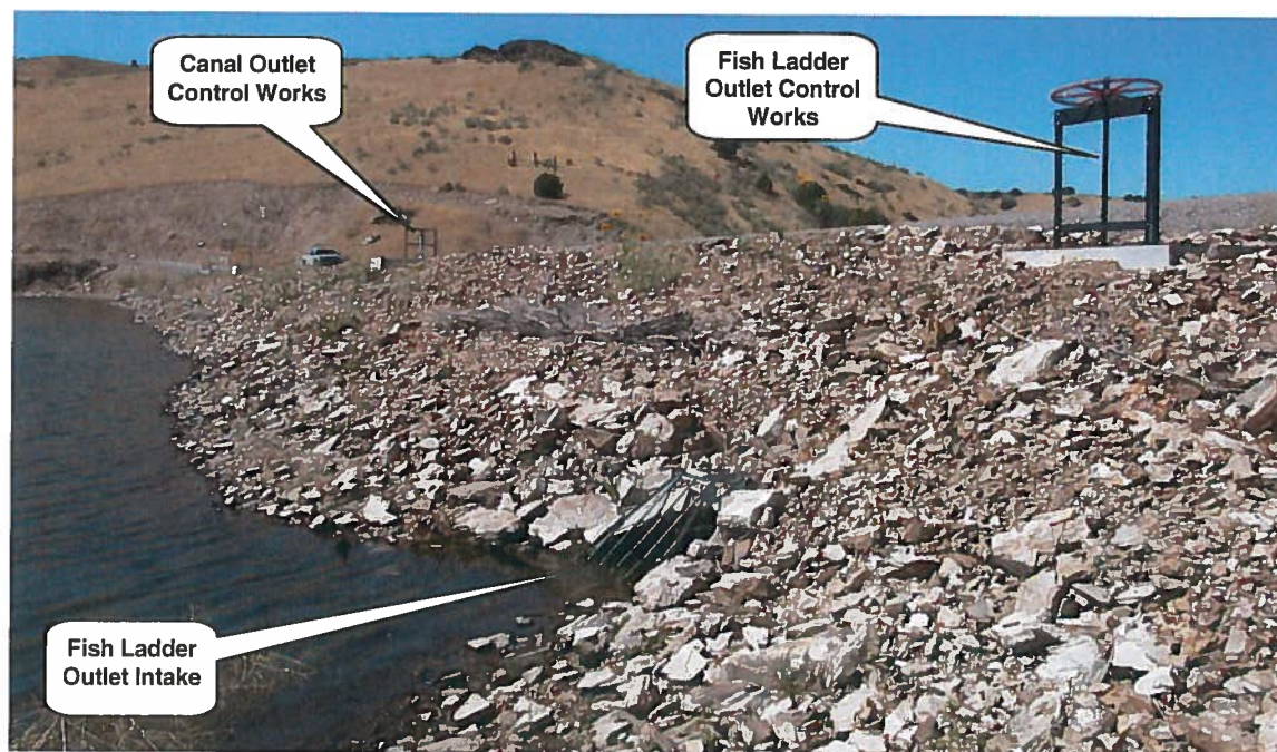
BELOW: View of the upstream slope of the dam from near the fish ladder outlet intake showing the reservoir level at the time of the inspection.
