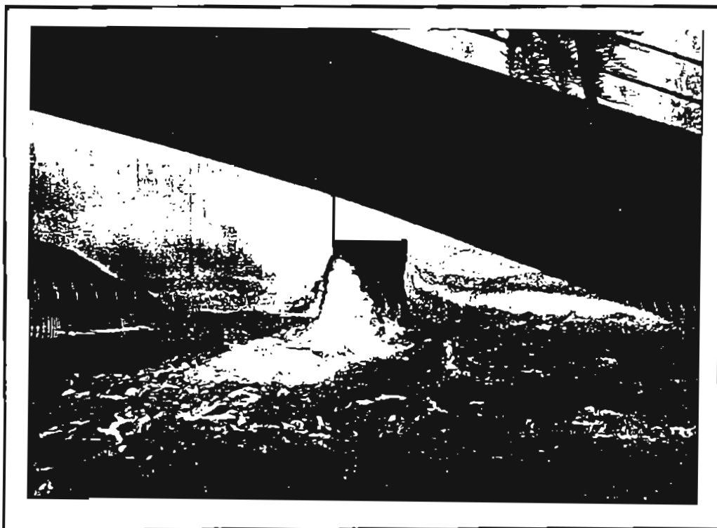
HOT WATER DISCHARGE INTO RIVER (UNDER BRIDGE)
