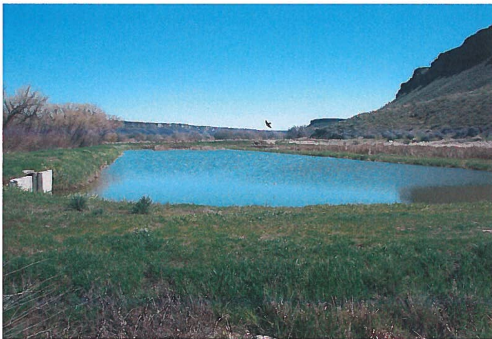
Figure 8: Deepwater pond and outlet
