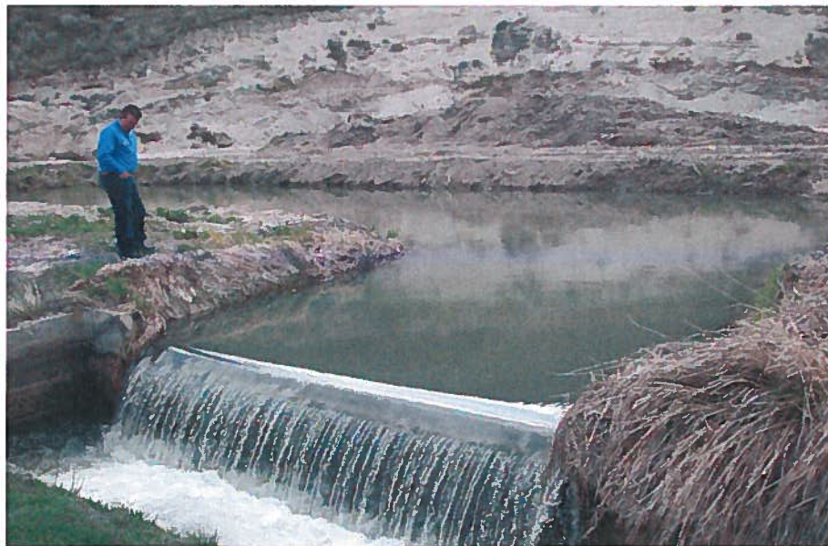
Figure 4: Contracted Rectangular Weir
