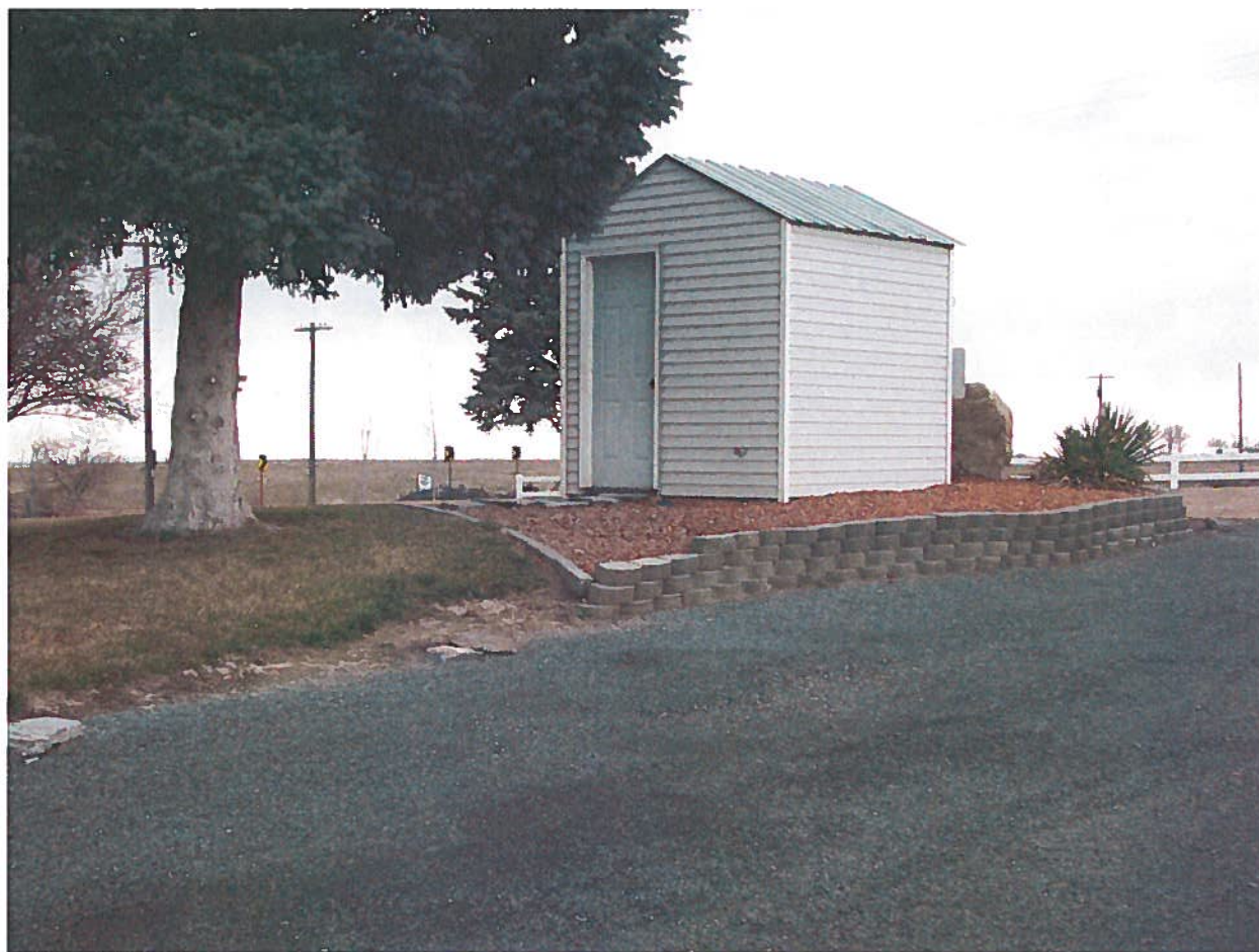
Figure 7: Well house on northeast corner of Deisher property. Supplies water for irrigation rights 47-17237, 47-17238 and 47-17239
