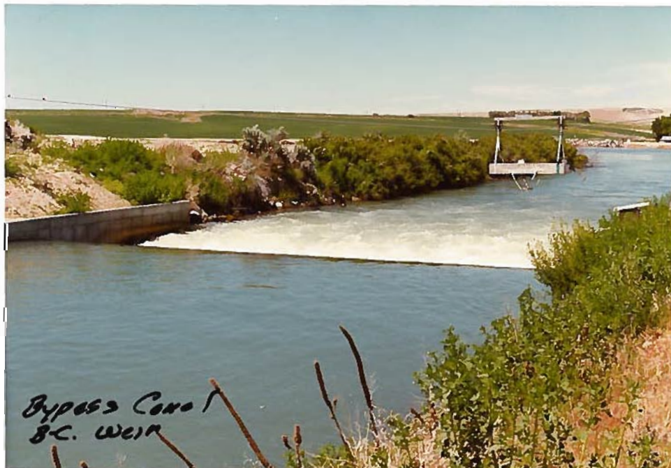
BYPASS CANAL BROAD-CRESTED WEIR
