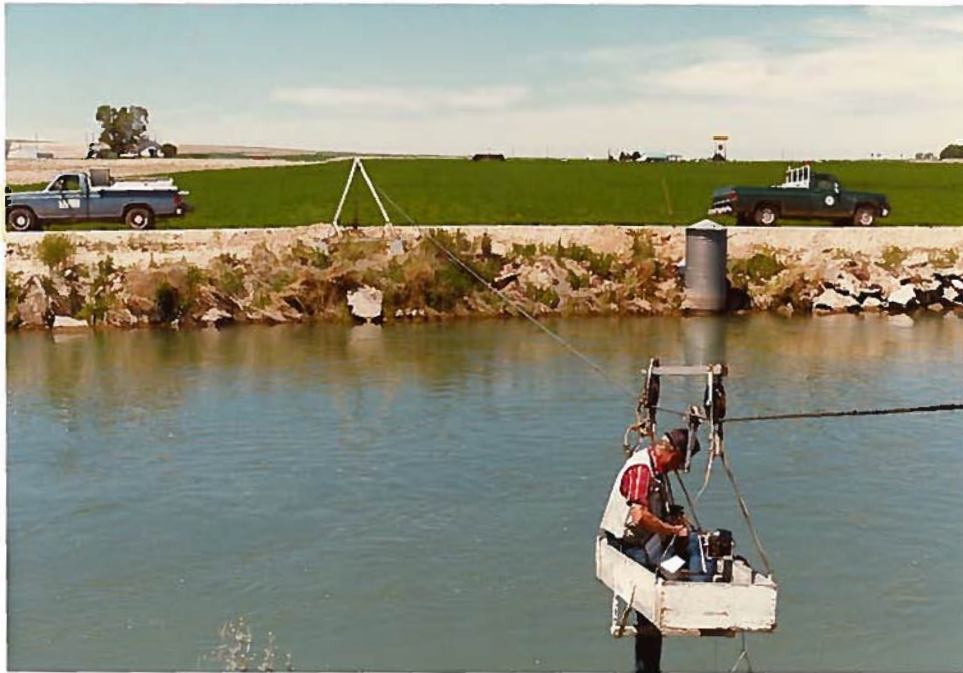
Outflow Gaging Station Main #2
