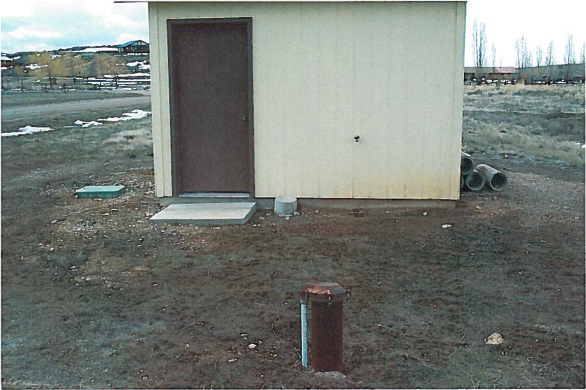
Well – Permit 37-20718 Looking West By J E Stanton 3-18-05
