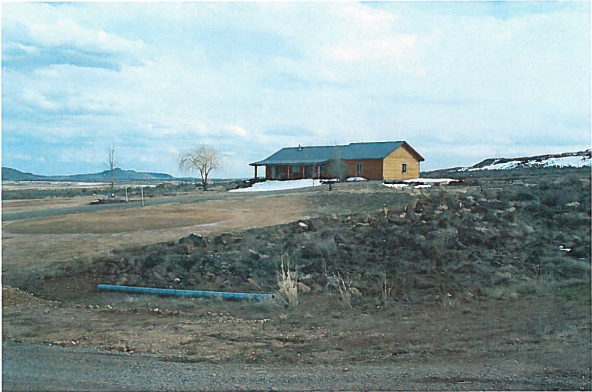
Home On South End of Property – Permit 37-20726 By J E Stanton 3-18-05
