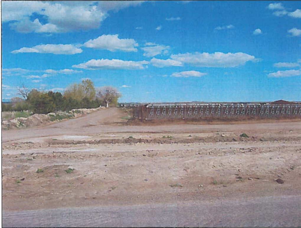
Figure 15: Place of Use at northwest corner facing east.
