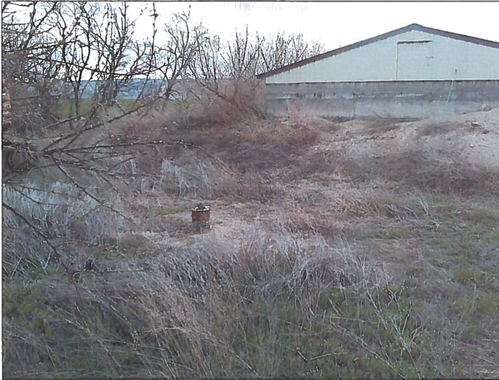
Figure 7: Well #4 and 50,000-gallon storage facility.
