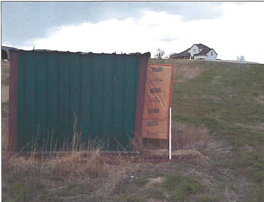
Figure 12: Well #7 pump house. The home in the background is also served by Well #7.
