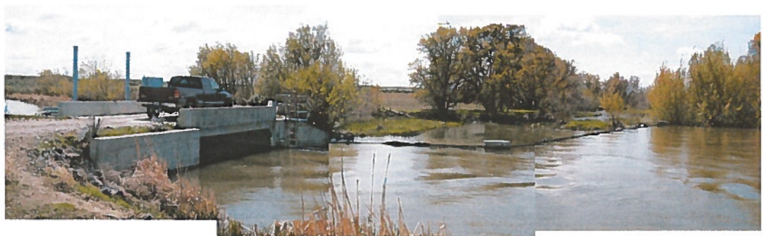
Downstream view of diversion dam.
