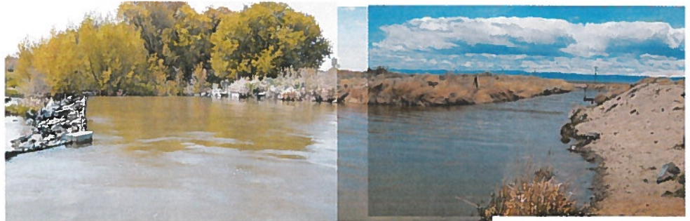
View of head of canal going to penstock.
