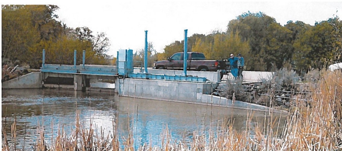
Upstream View of diversion.
