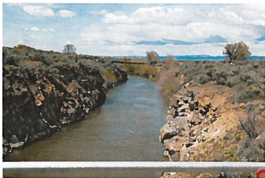
Excavated channel below power plant leading back to Little Wood River. View looking downstream.
