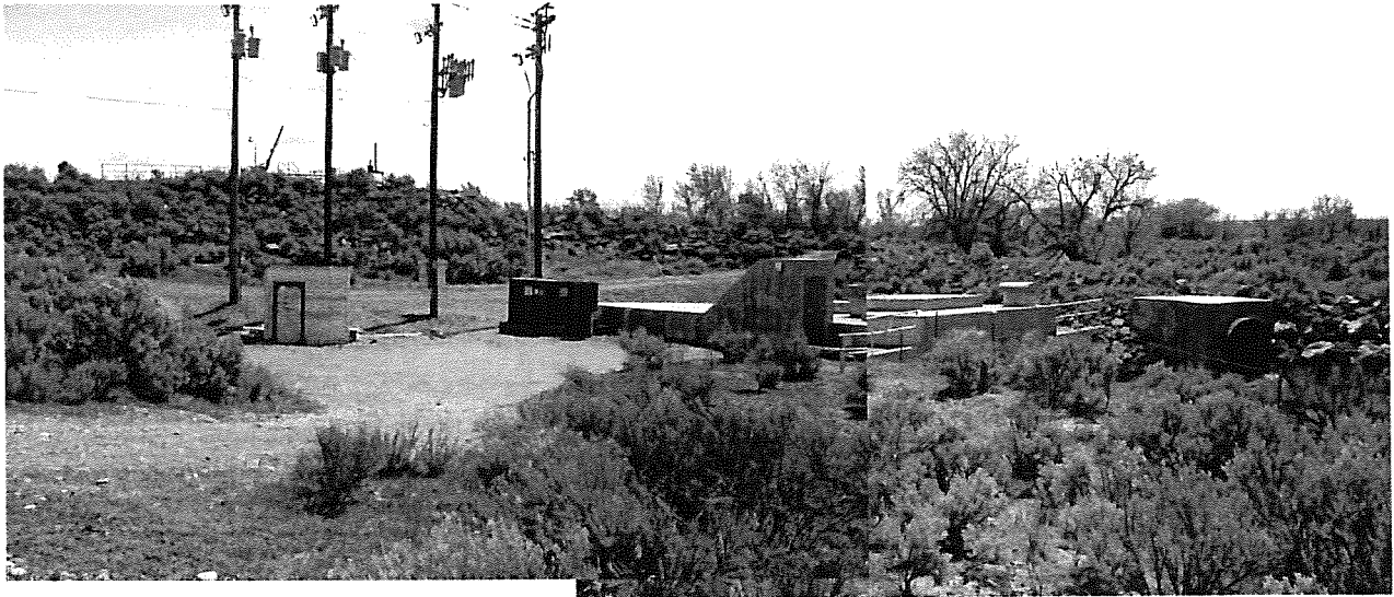
View of power plant from right bank. Head of penstock in background.
