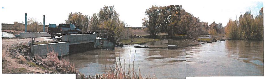
Downstream view of diversion dam.
