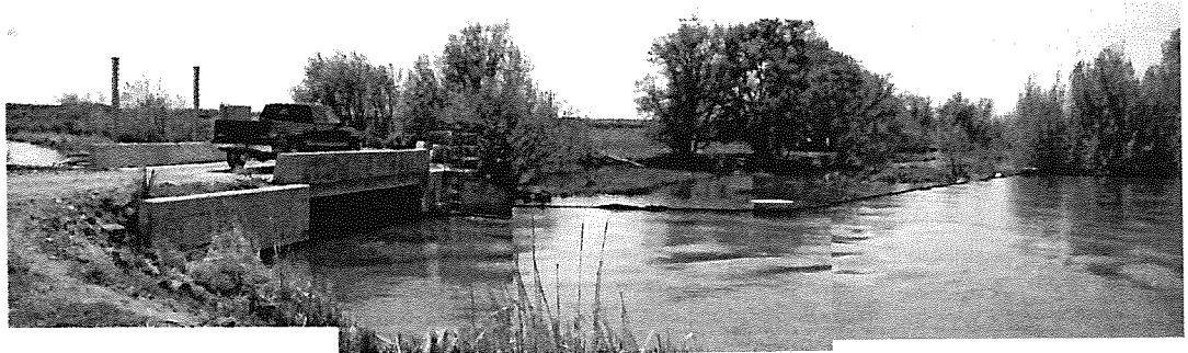
Downstream view of diversion dam.
