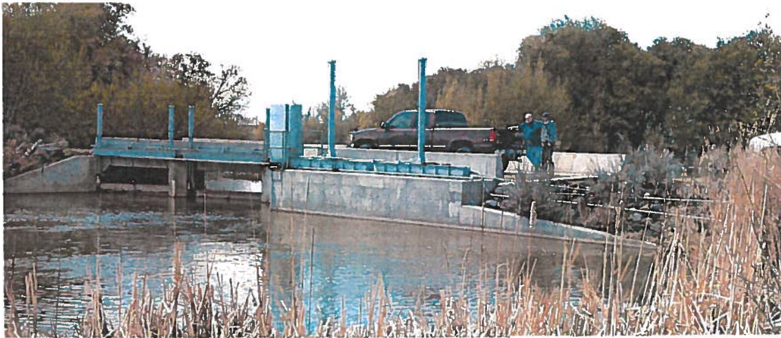
Upstream View of diversion.
