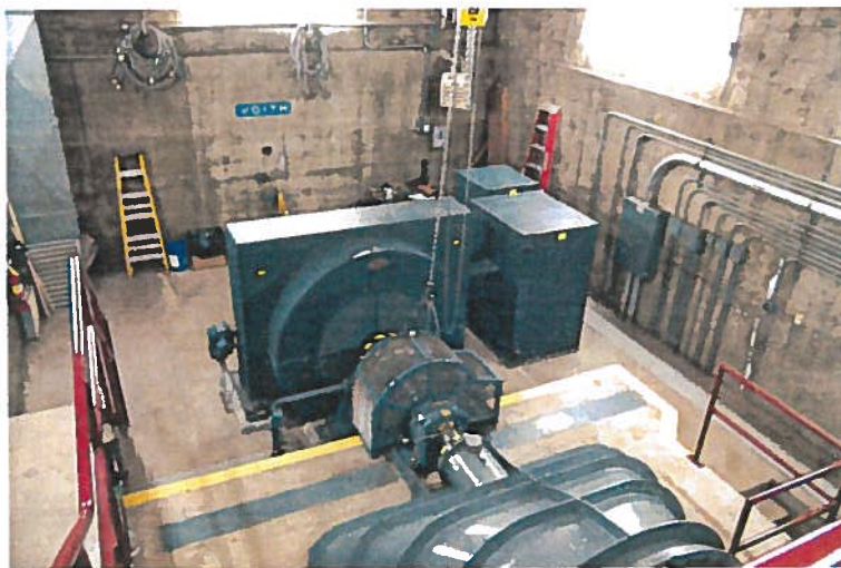
View taken from control deck looking downstream from within power plant.
