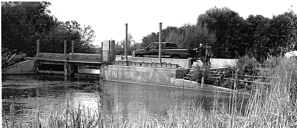
Upstream View of diversion.
