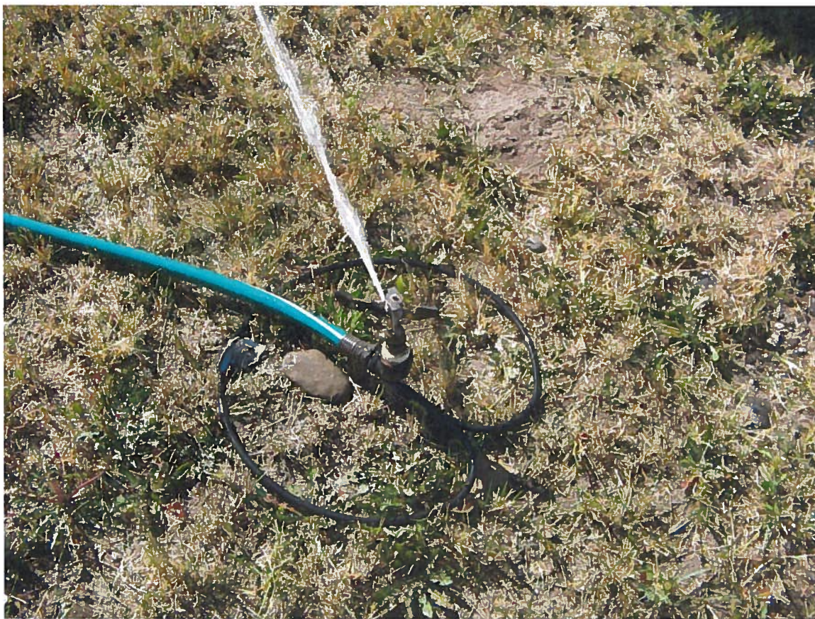
Picture of one of the Rain Birds in operation.
