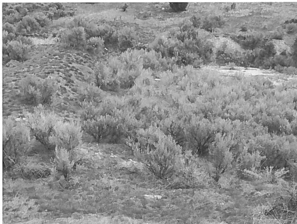
Figure 4: Earthen Dam on lower reservoir
