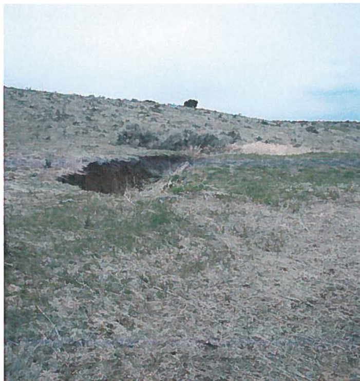
Figure 2: Upper reservoir spillway
