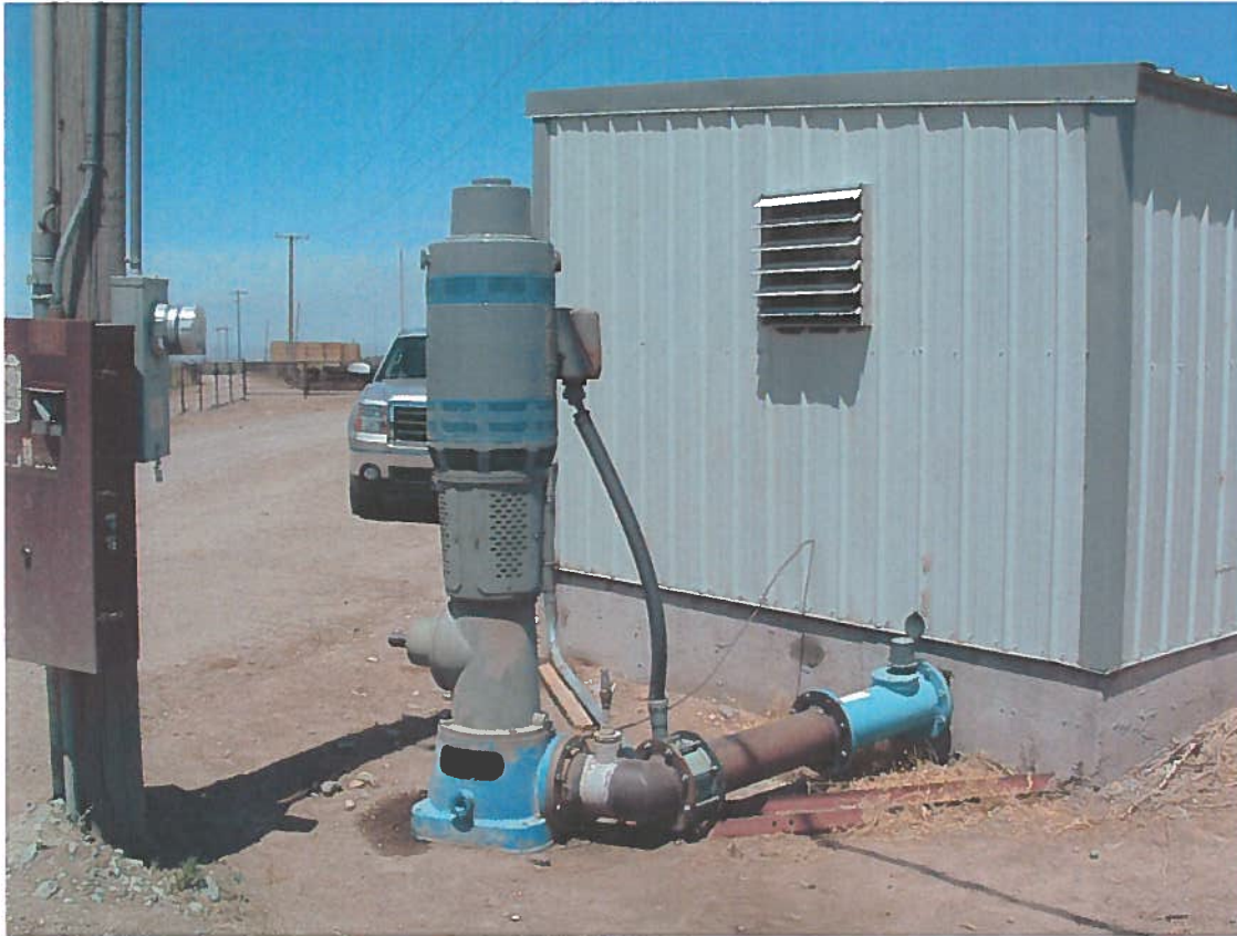
Well 1 (Feedlot Well) – 125 hp pump
