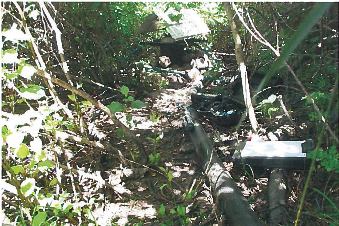
Upstream view of delivery pipe and plant.
