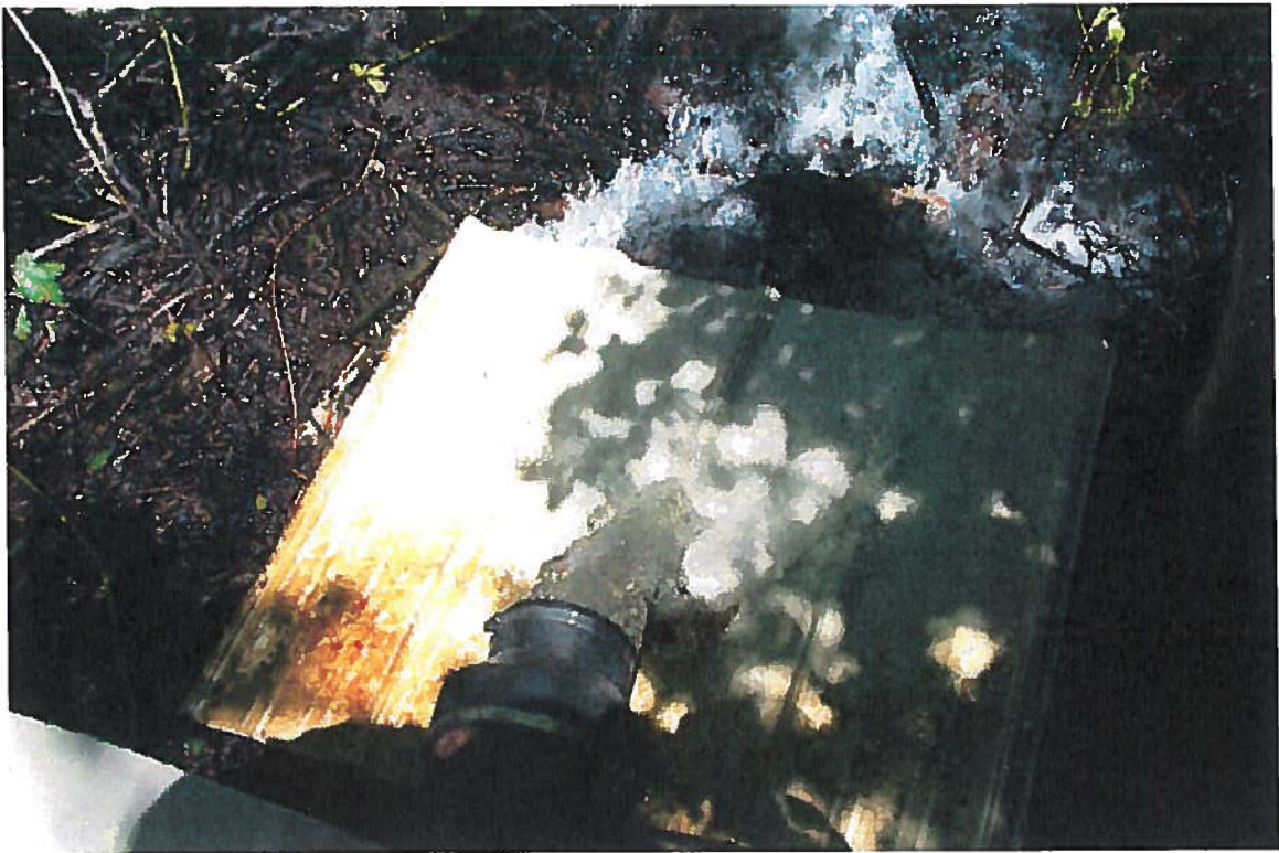
Water Discharging from Hydroelectric Generator Back into Lower Rock Creek
