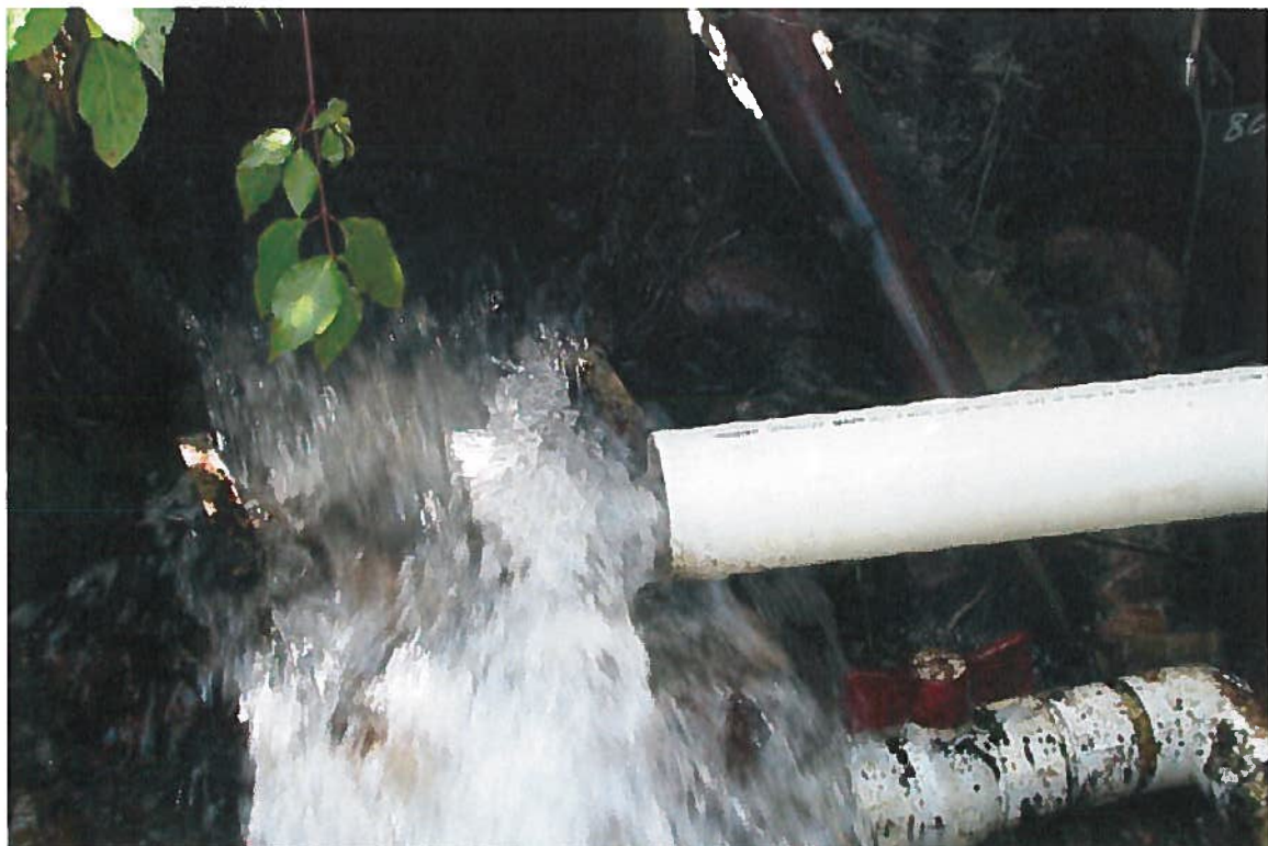
Close-up view showing regulating valve on pipe.
