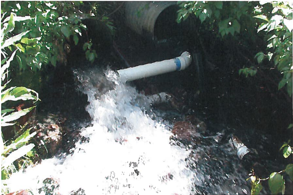
Penstock and pipe inlet at County road culvert outlet.
