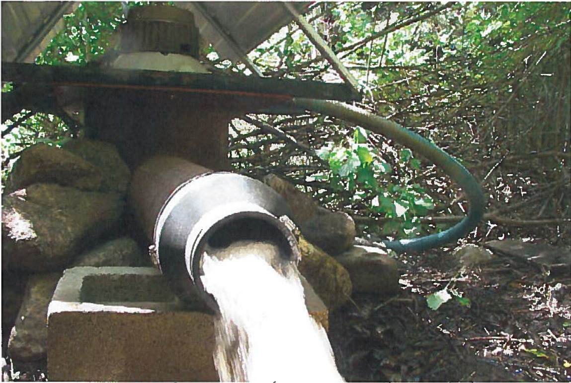
Hydroelectric Generator (Background) and Discharge pipe.
