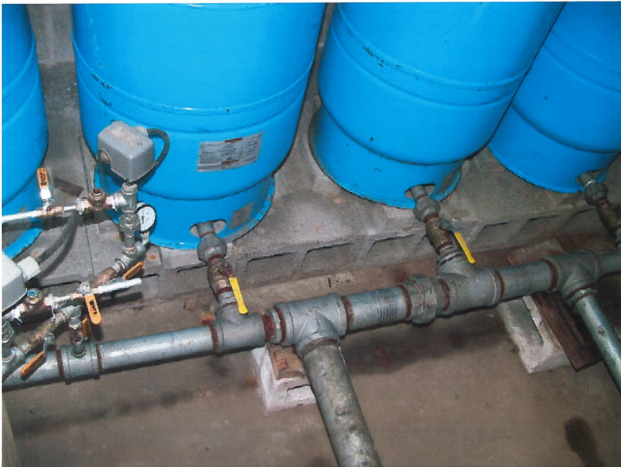
Space Across Plumbing in Well house
