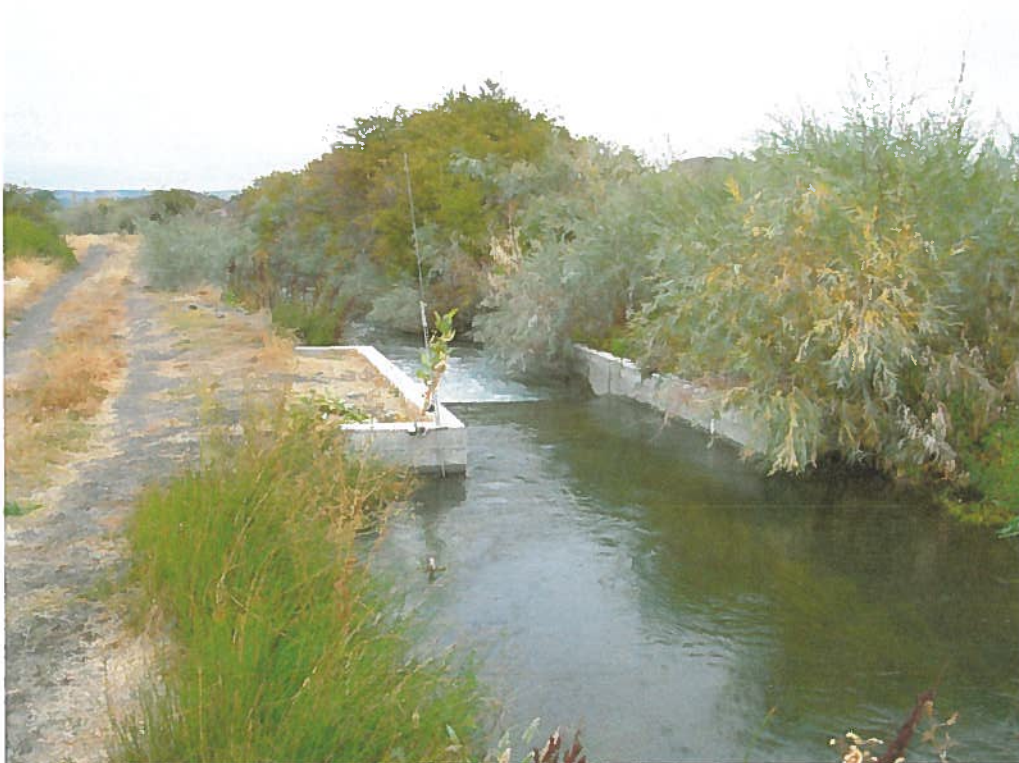
Looking Downstream at Weir About 75 Feet Below Gates
