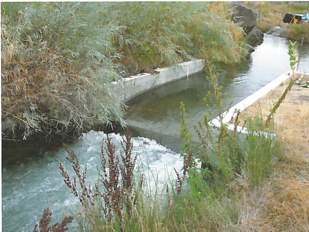
Looking Upstream at Weir
