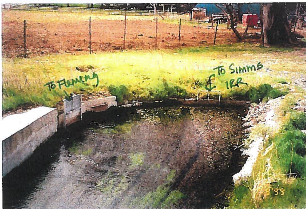
Settling Pond Below Lower Pond (Looking West)
