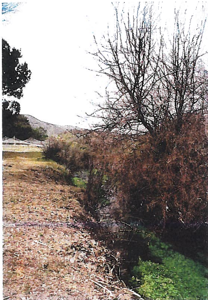
Ditch To Upper Ponds (Looking SW)
