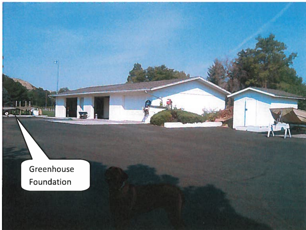
Figure 6: Eastman Garage/Shop & Greenhouse Site
