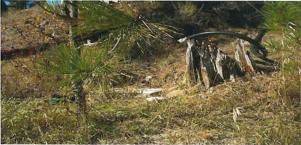
Point of diversion location – cement slab where pump is located when in use. Also see 1.5 inch pvc pipe that pushes water up hillside (approx. 20 feet of lift) to place of use
