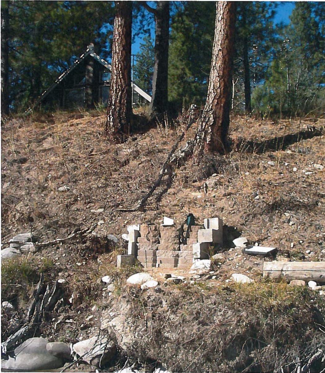
Point of diversion on river bank – pump is anchored at this point when in use (pulled for winter and in garage) – Note 1.5" pvc pipe that pushes water up to place of use (lift is approx. 25')
