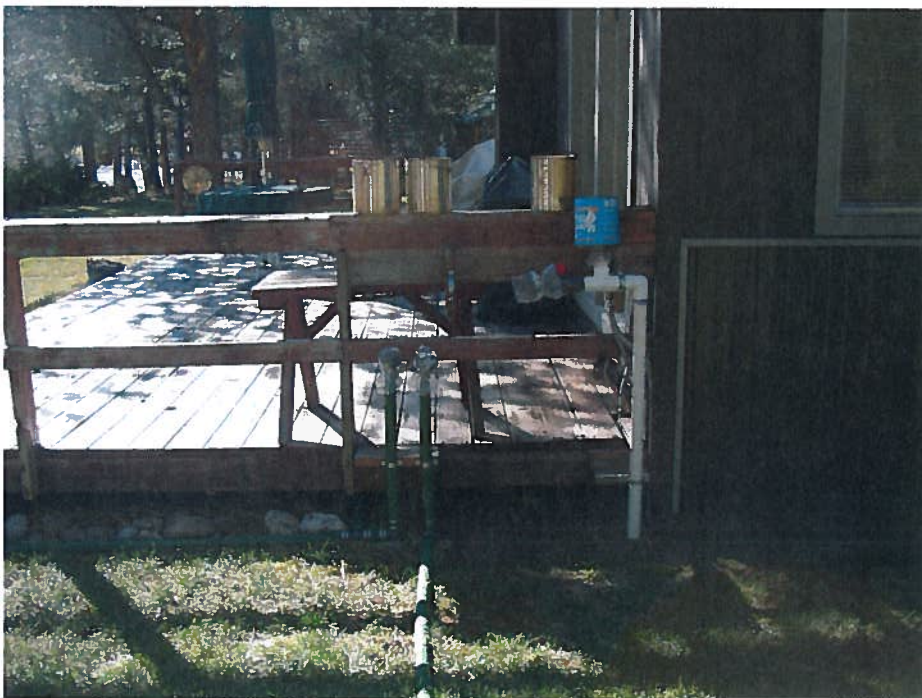
Point where sprinkler lines are routed to "zone 1" or "zone 2" (see map attached showing zones) when in use
