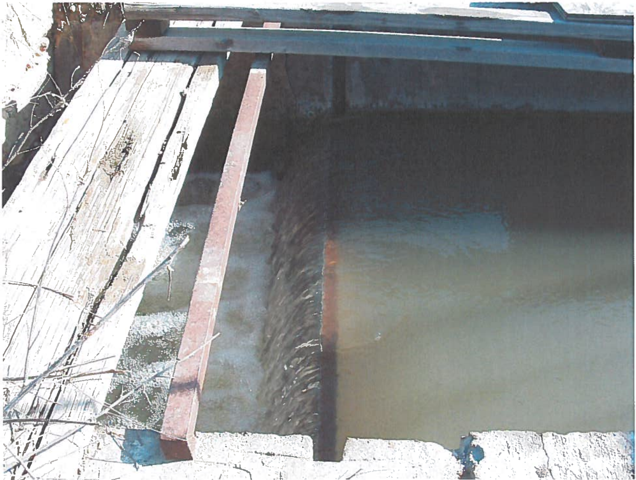
Flow over weir at 2 cfs +/-
