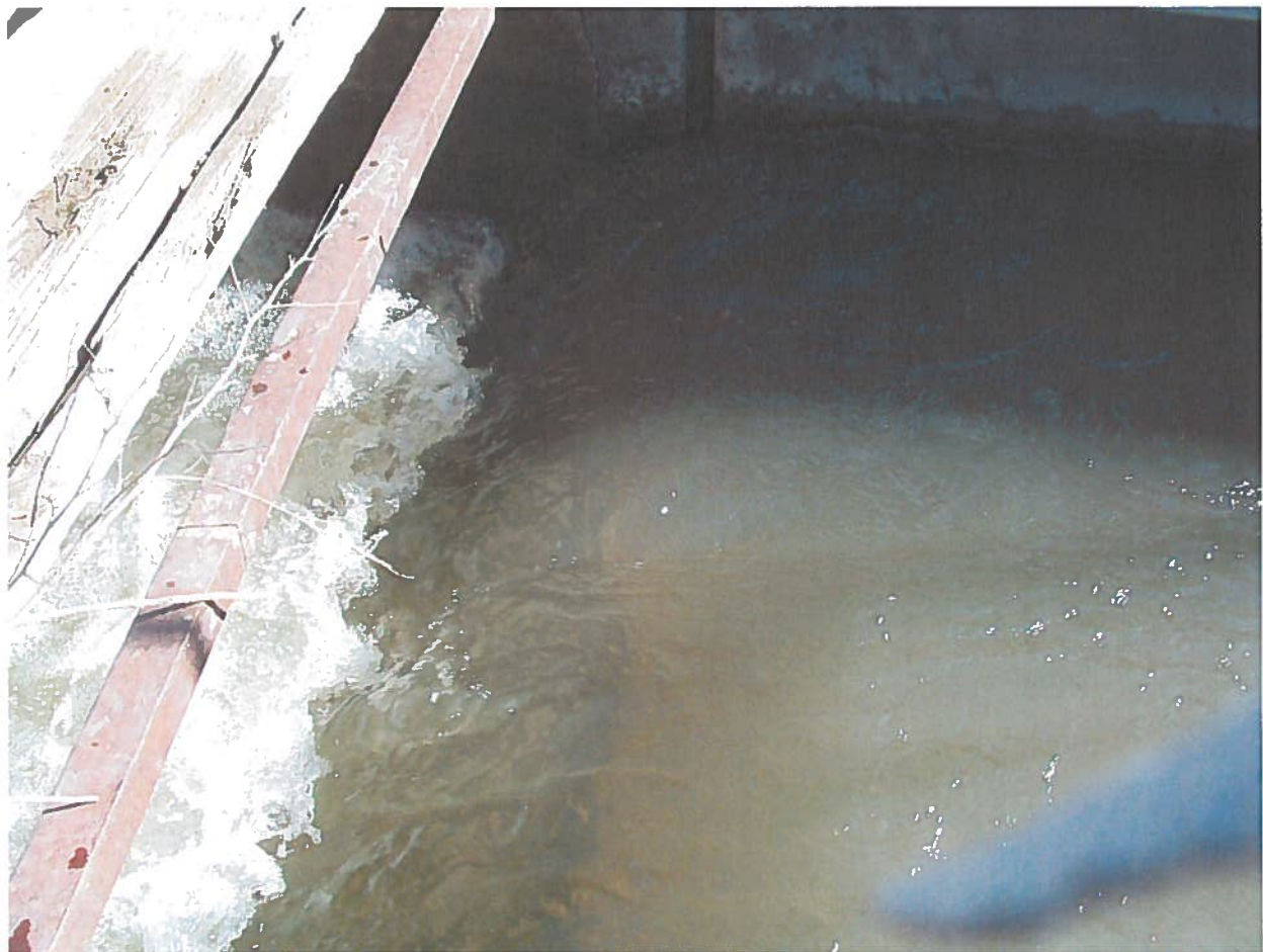
Flow over weir at 7 cfs +/-
