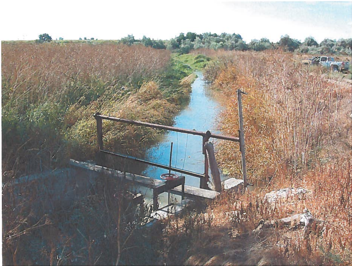
Baldridge and Meadows Drain with check structure in the foreground. Diversion for Upper Haas Ditch is out of sight near pickup truck in background.
