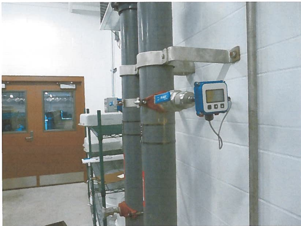
Figure A6: SeaMetrics meter on CGW in incubation room
