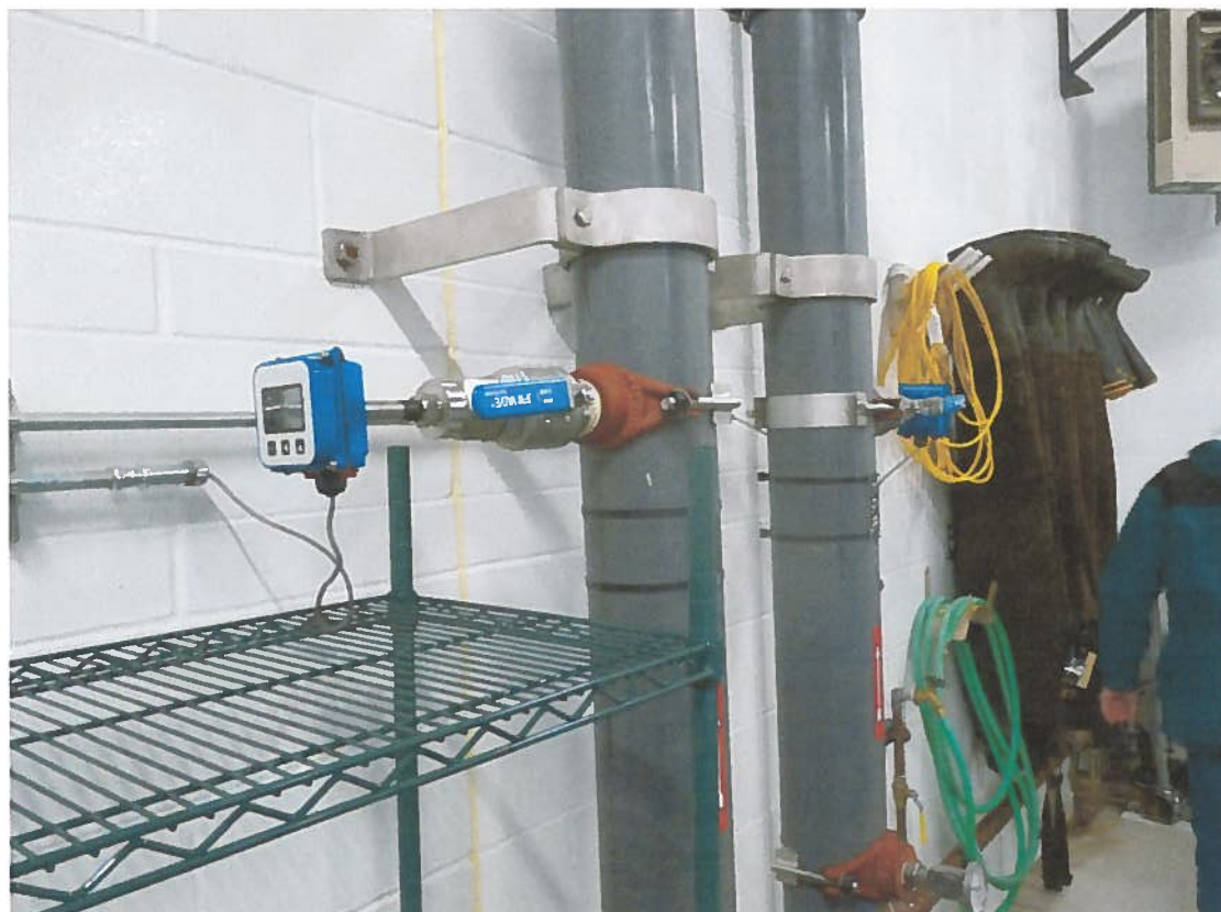
Figure A5: SeaMetrics meter on AGW in incubation room.
