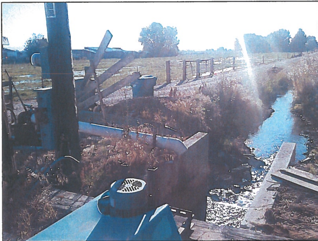
Photo showing McMullen Lateral and discharge pipe. Well is on left.
