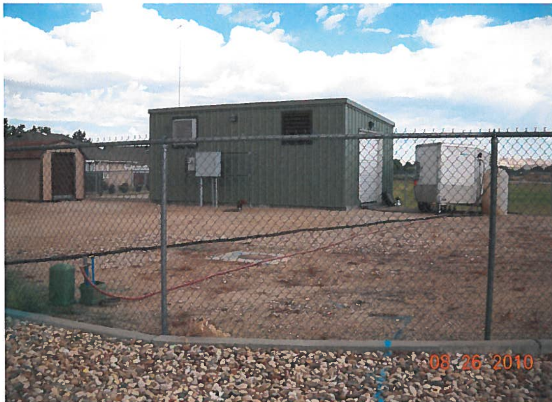
Wellhouse north of 12 th Street and southwest of Carberry School. Well is located just inside the white door seen at end of building.
