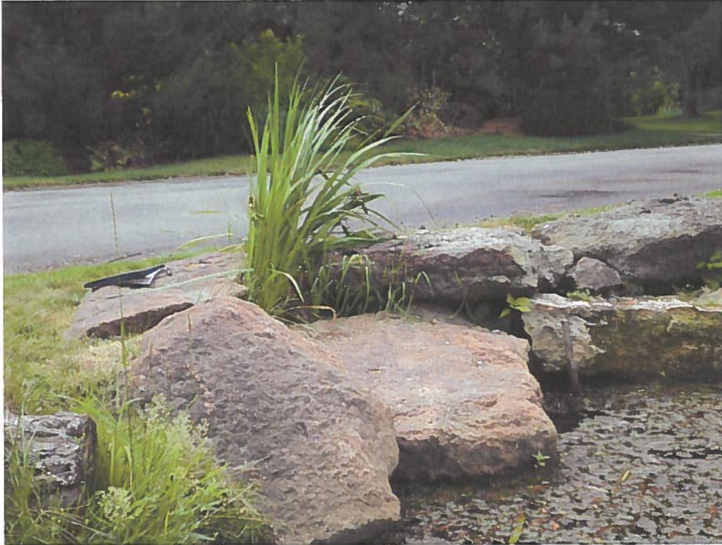
Photo 3: Pond 4 looking SE, culvert running under Lakemont Dr.
