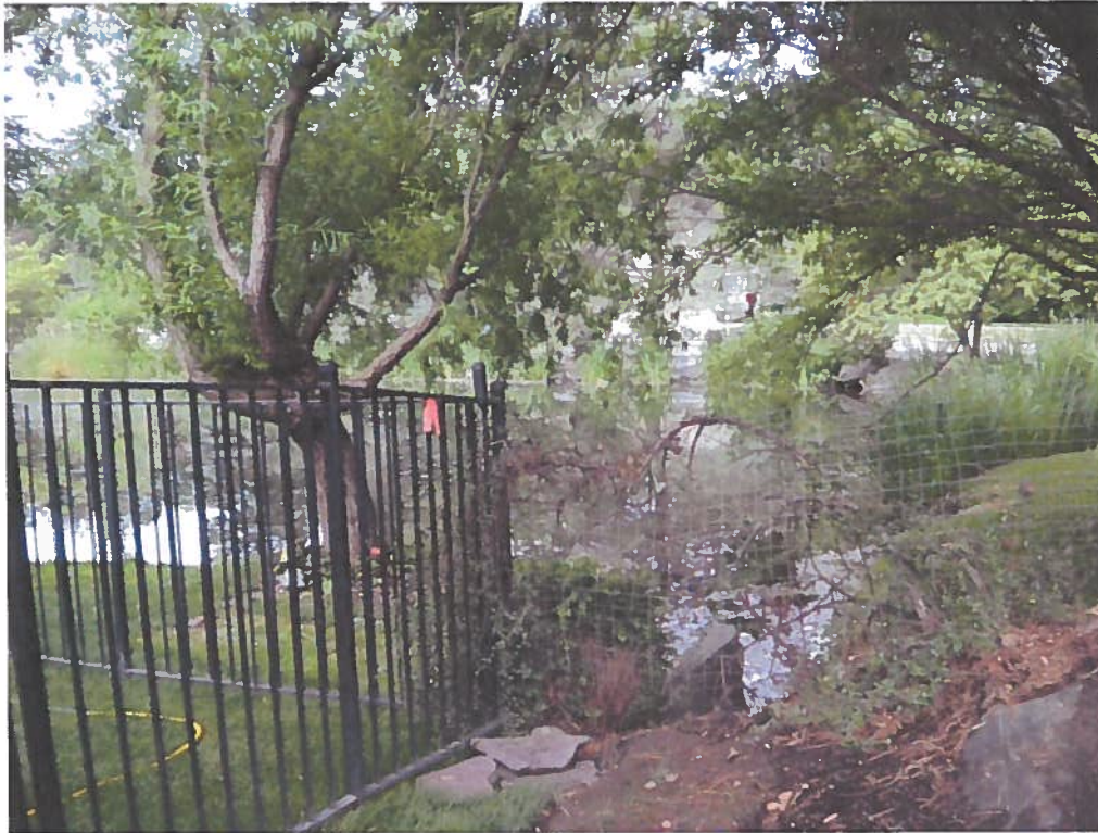
Photo 5: Pond 3, looking SW from NE edge; culvert in photo is an outlet to another pond to the west of subdivision
