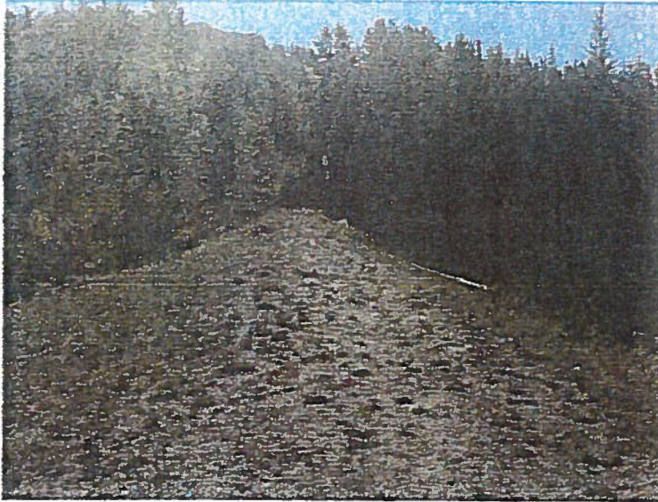
Dam crest standing on northeast end near spillway and looking southeast
