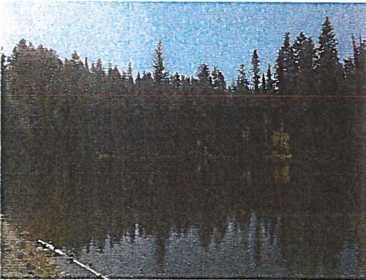
Reservoir looking straight south from northeast end of the dam
