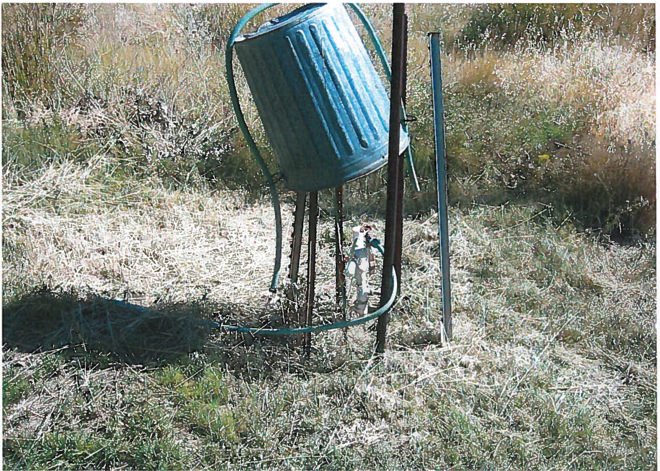
Outlet of underground pipe at POU.
