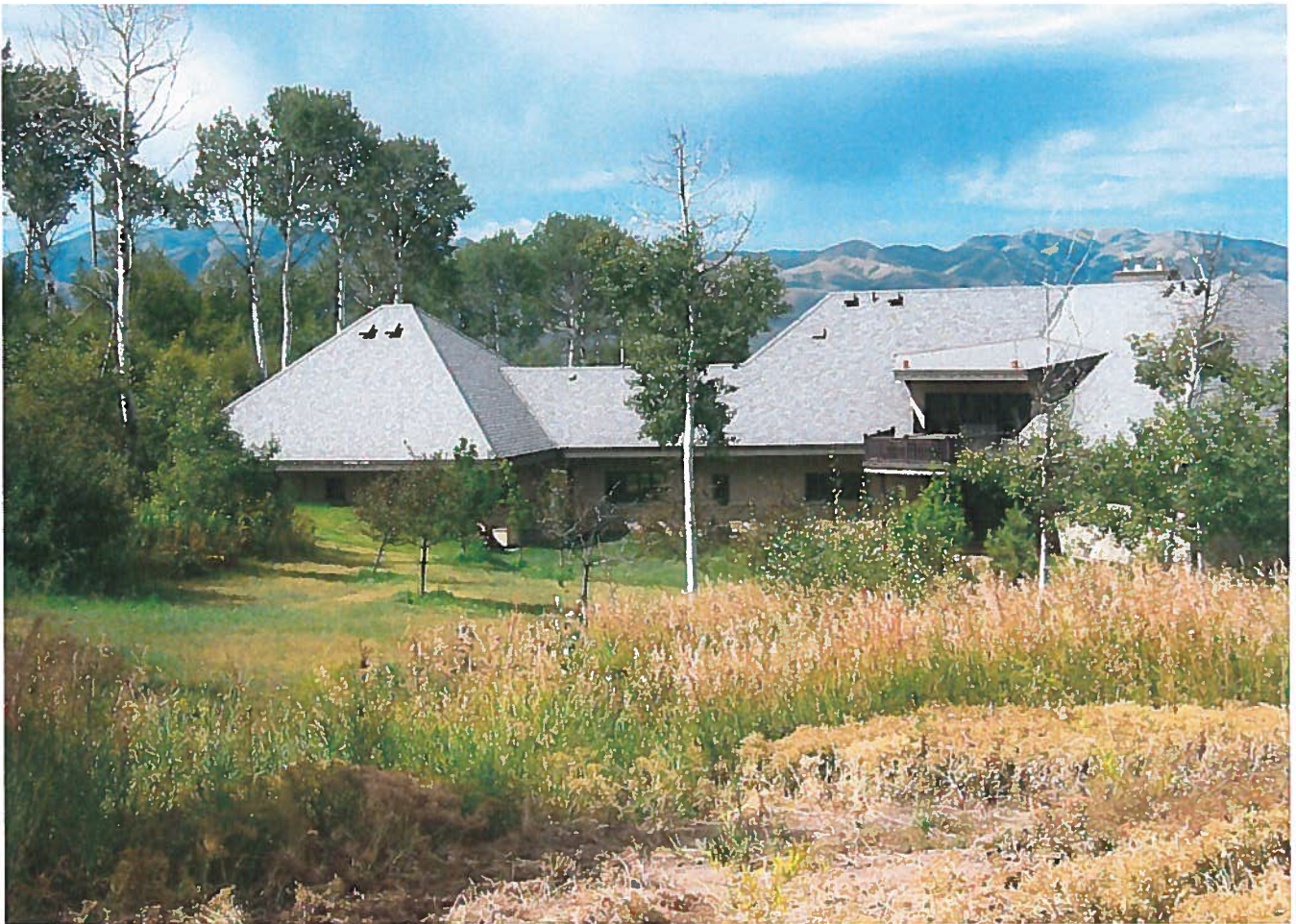
Nestor Home From Cistern Area
